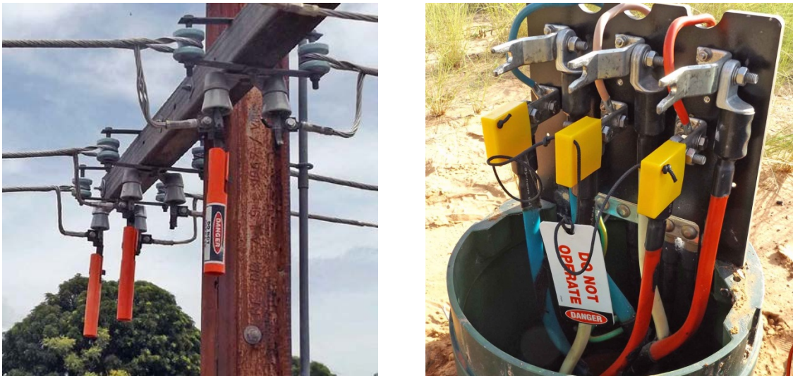
Figure 3-31 Examples of barriers for disconnectors
