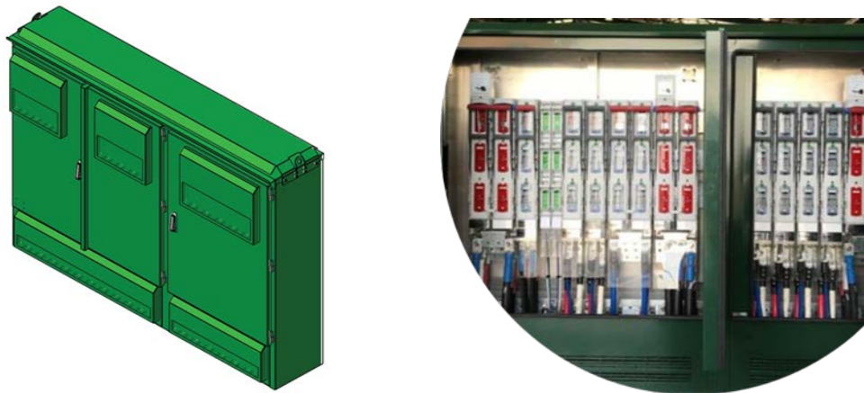
Figure 3-22: Type 3.1 Kiosk rated at 2800A/415V
