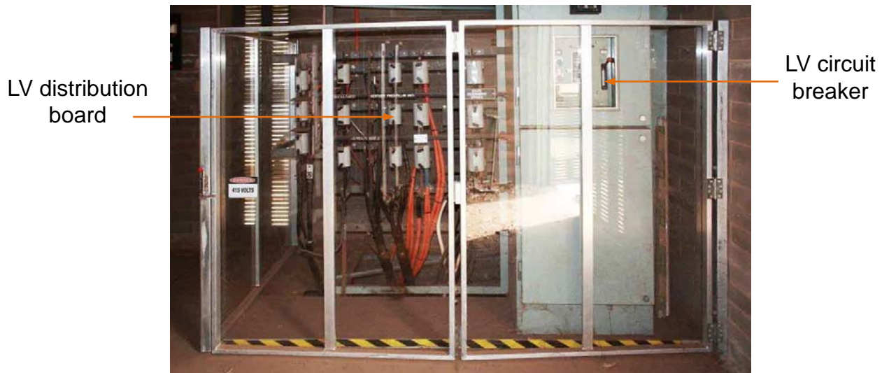
Figure 3-15 Distribution board mounted disconnectors (hinged)
