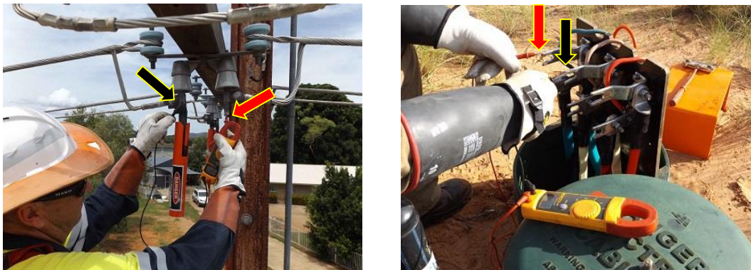
Figure 10-6 Phasing LV disconnectors
