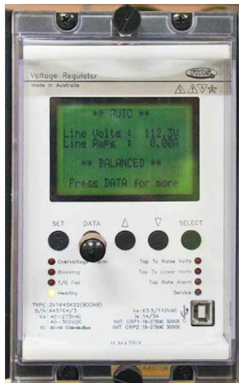
Figure 6-33 Typical AVR relay
