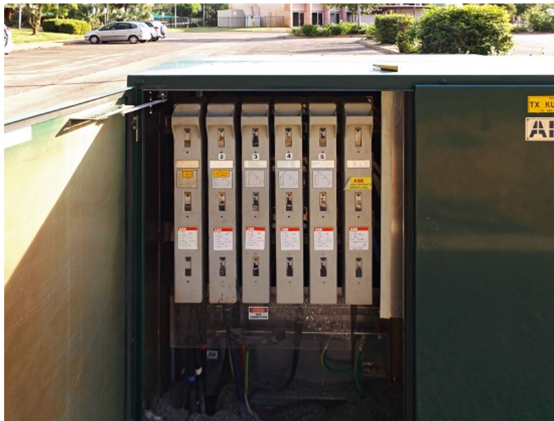
Figure 3-14 Distribution board mounted disconnectors (extractable)
