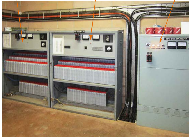
Figure 6-27 Typical battery chargers and banks
