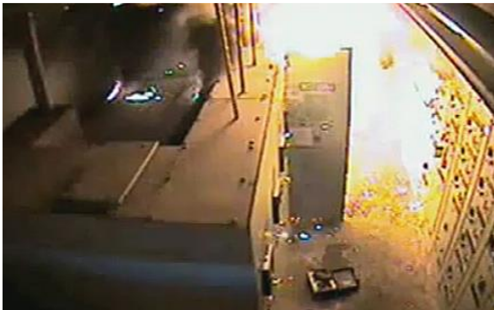
Figure 8-25 Indoor switchboard arc flash and arc blast
