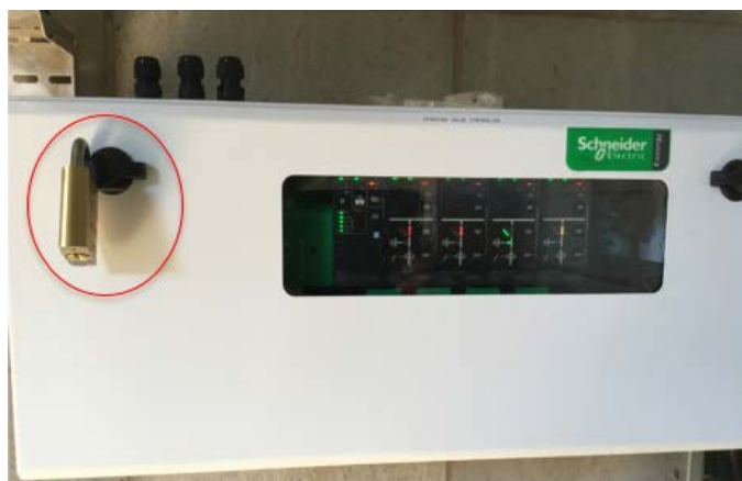
Figure 5-13 T300 Locked Enclosure.
