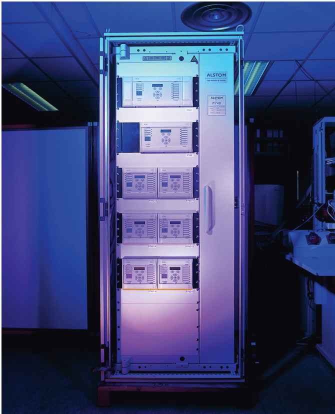
Figure 15.21: Busbar protection relay using the latest numerical technology (MiCOM P740 range)
