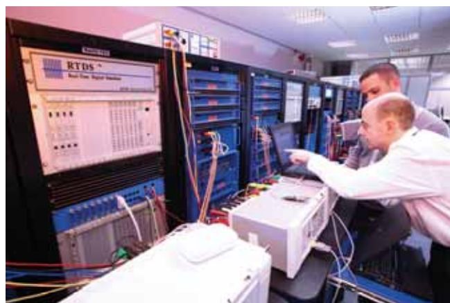
Figure 21.12: Digital power system simulator for relay/protection scheme testing
