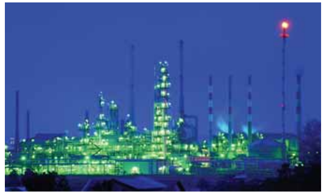
Figure 18.1: Large modern industrial plant
