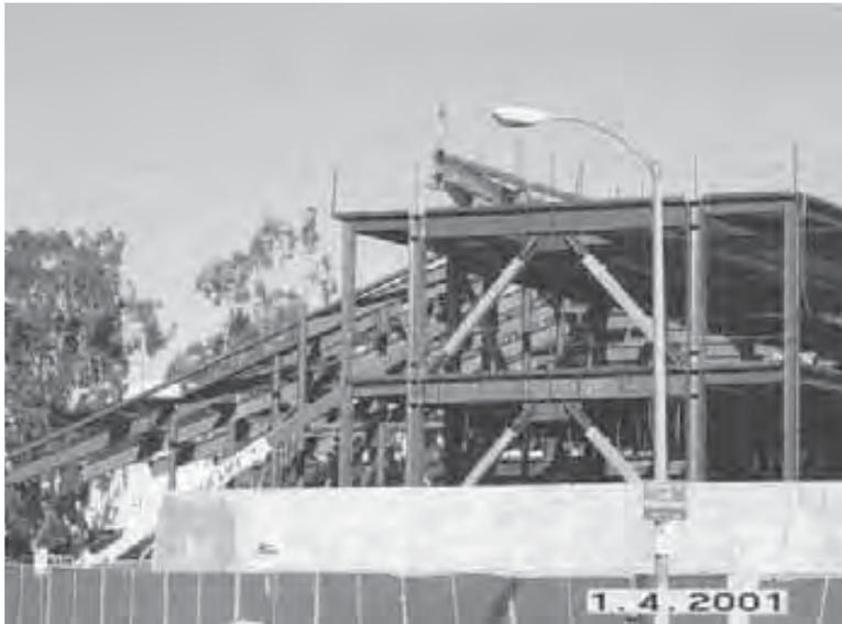
**Figure 8.36d.** Unbonded brace frame elevation.
