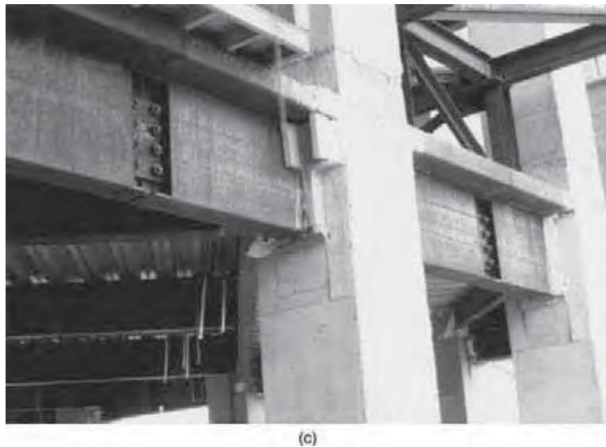
**Figure 5.13.** Composite tube with steel spandrels: (a) typical floor plan; (b) typical cross section through spandrel; (c) detail at perimeter column and spandrel intersection.
