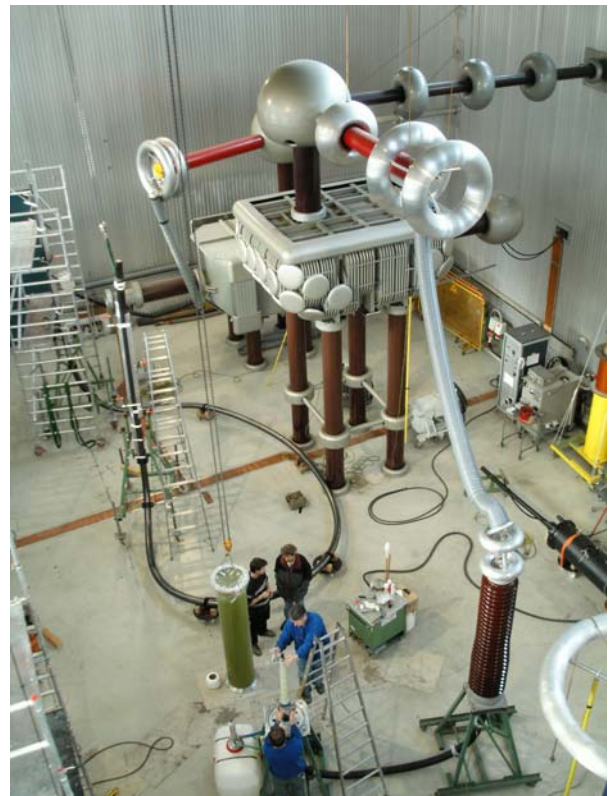
Picture 9: Sample test of stress cone in Sefag ixosil high voltage laboratory
