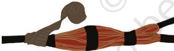
Fig. 5.10 Wrapping the cable with mesh tape
