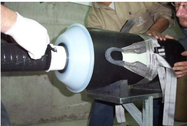
Picture 11: Installation of a 245kV joint supervised by instructor
