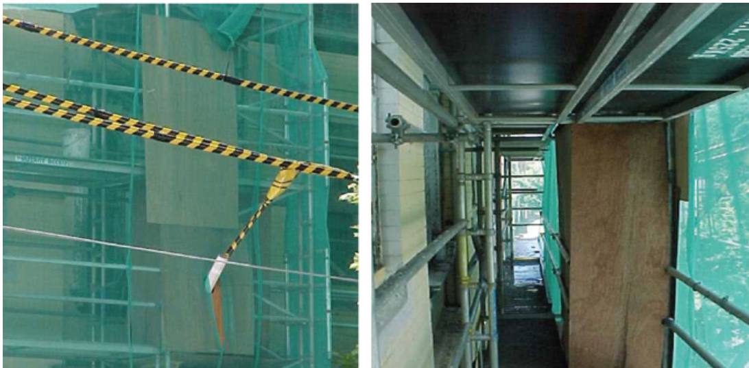
Figure 11 – Enclosure of overhead powerlines
