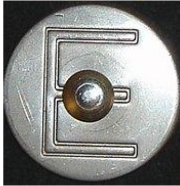
Figure 13: Approved kerb marking
