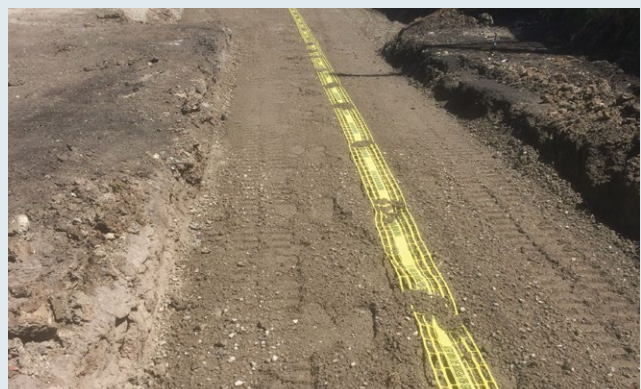
Figure 24: Yellow marker tape in a trench to provide warning of underground gas services
