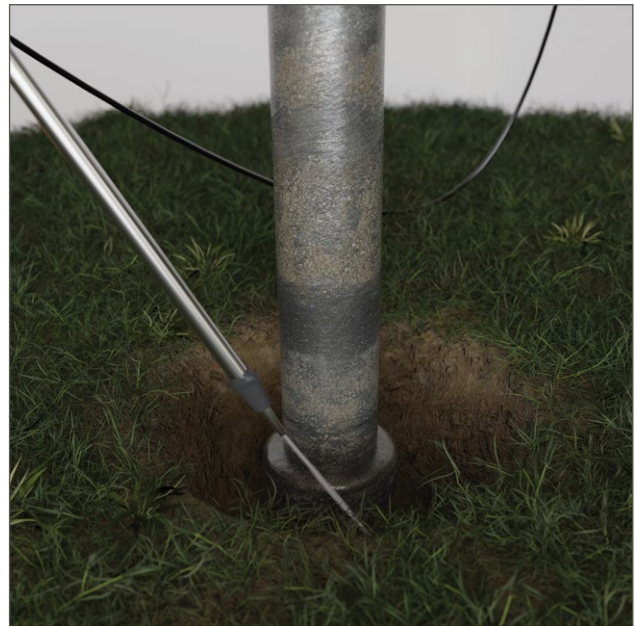
Figure 20: Two images showing the potholing technique
