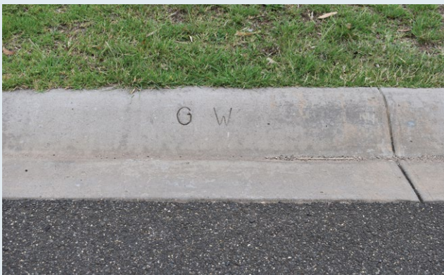
Figure 13: The markings "GW" (stands for Gas Water) on concrete guttering indicates gas and water assets beneath.
