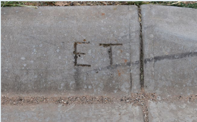
Figure 7: The markings "ET" (stands for Electrical Telecommunications) on concrete guttering indicates electricity and telecommunication assets beneath.
