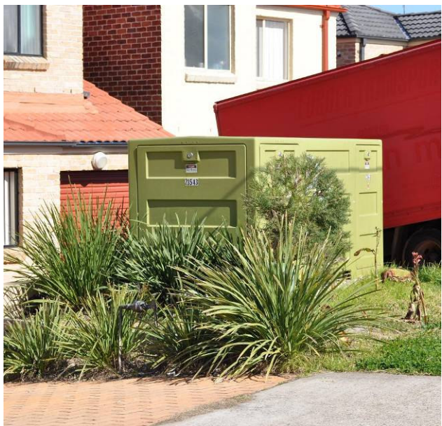
Padmount substation (above) and pole mounted substation (right)
