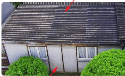
Fibro-cement asbestos sheeting
