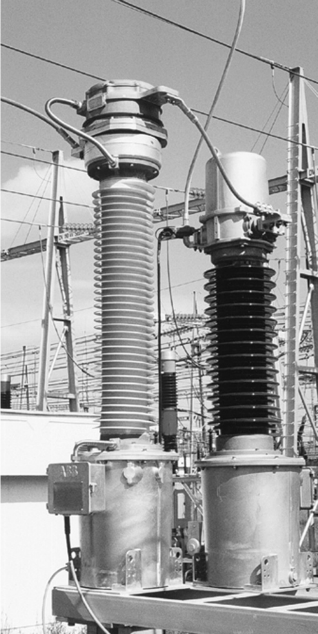
Figure 5.7 Optical CT HV installation (courtesy of ABB)
