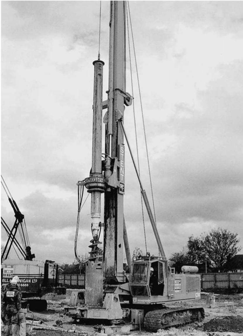
Figure 15.5(b) Auger for forming cast- in-situ concrete piles – 400 kV Sellindge substation, Kent
