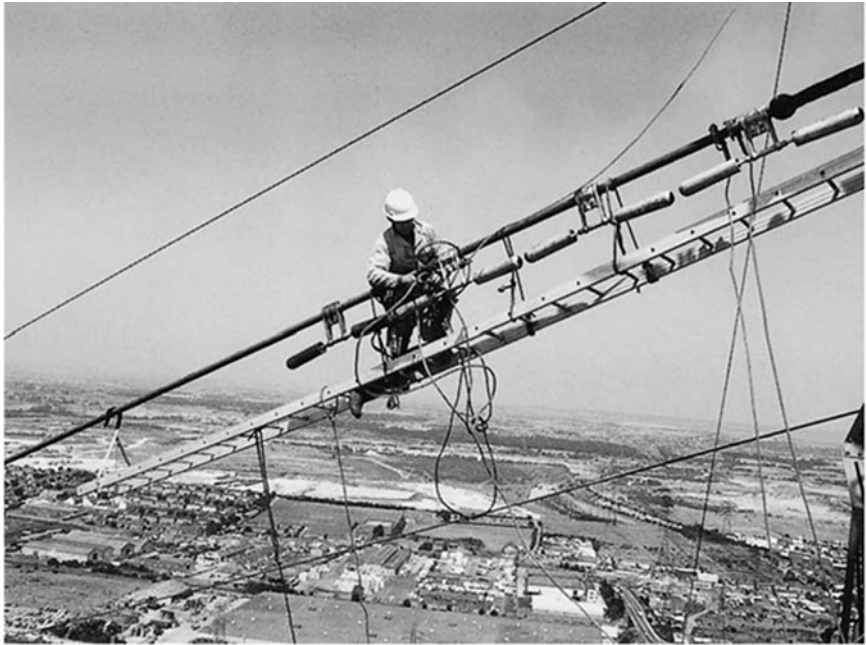
Figure 18.19 Vibration damper replacement, 400 kV Thames crossing reinsulation
