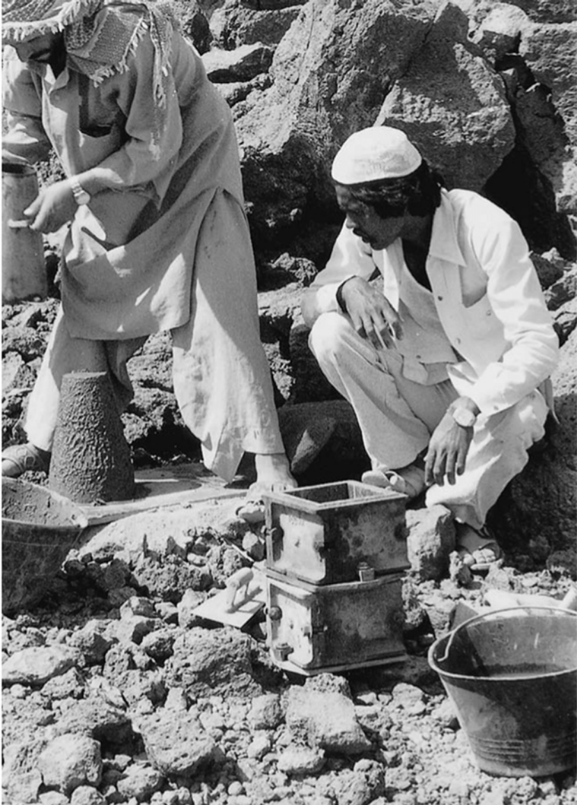
Figure 15.8 Concrete cube and slump cone samples being prepared –Yanbu-Medina 380 kV transmission line, Saudi Arabia (courtesy of Balfour Beatty Projects and Engineering)
