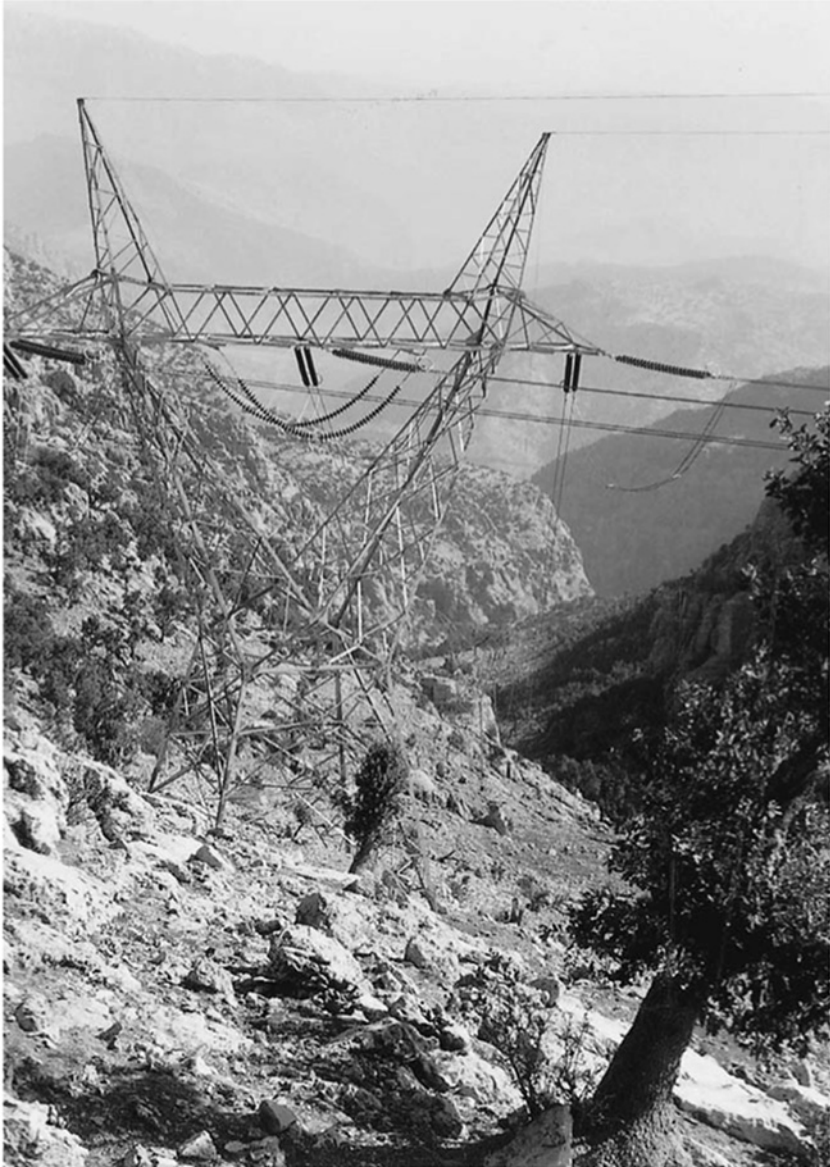
Figure 16.2 400 kV single circuit twin conductor overhead line crossing the Zagros Mountains in Iran (courtesy of Balfour Beatty)
