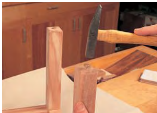
Small plastic furniture glides are simply nailed in place.
