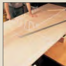
36 Laying Out and Cutting Plywood
