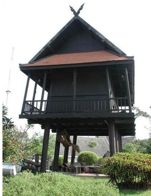
Fig. 1. Traditional Thai House (single type) in central region [3].
