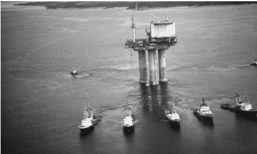
FIGURE 6.4 Towing concrete platform out of Norwegian fjord. Note small tugs pulling astern in order to provide control. (Courtesy of Aker Maritime.)
