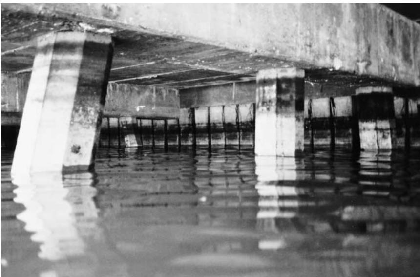
FIGURE 4.13 Example of durable concrete after 30 years exposure, Kuwait.
