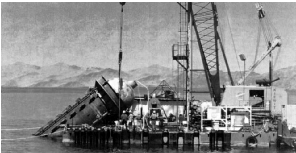
FIGURE 10.8 Installation of steel casing into pre-drilled shaft in 200 ft. of water, Lake Mead, Nevada. Note spacers to maintain annulus for tremie concrete infill. (Courtesy of Southern Nevada Water District.)
