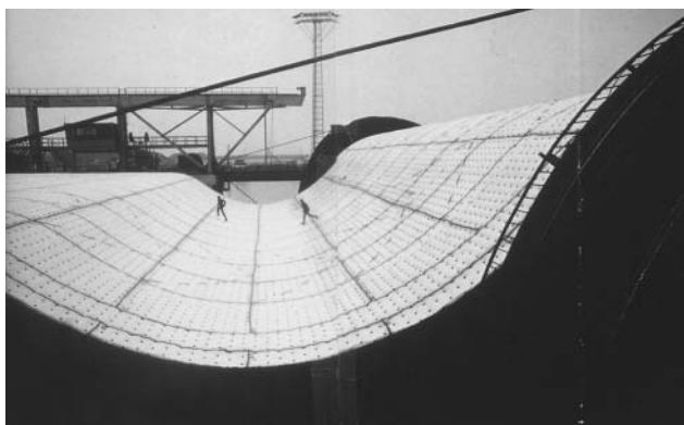
FIGURE 9.61 Rolling-up foundation mattress for transportation to site where it will be laid to prevent erosion of seafloor by strong tidal current and waves. (Courtesy of Ballast-Nedam.)
