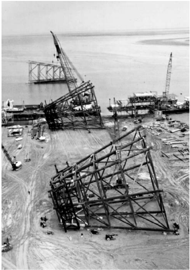
FIGURE 10.21 Prefabricating jackets for offshore terminal, Kharg Island, Iran.
