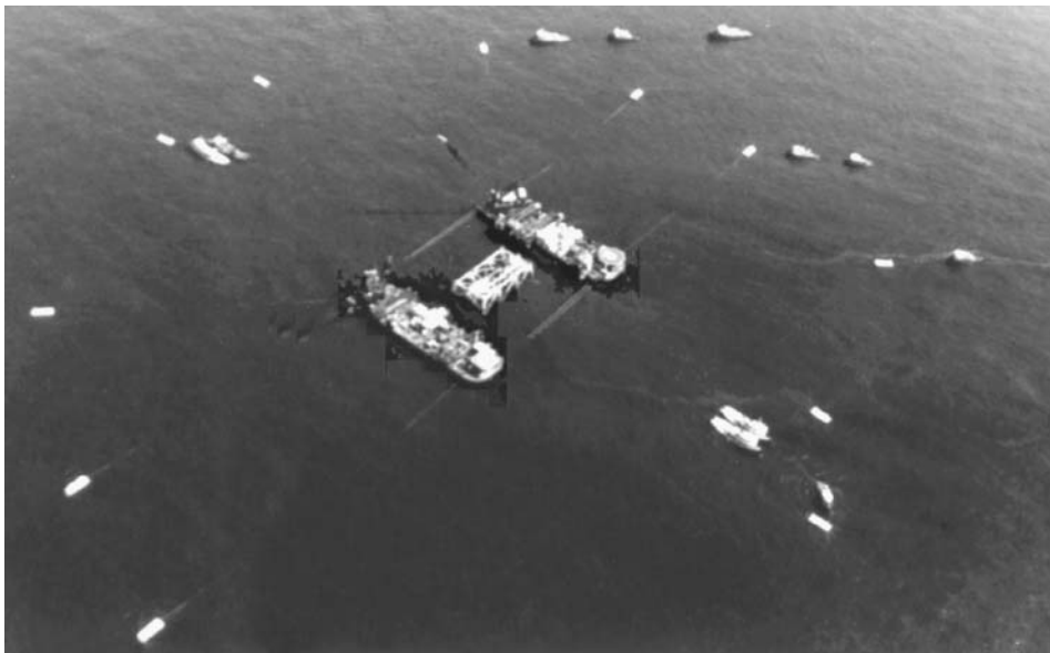
FIGURE 11.35 Mooring buoys and crane barges for assembly of Cognac jacket. (Courtesy of Shell Exploration and Production.)
