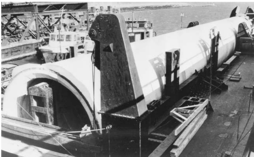
FIGURE 9.41 Transporting pile for Oosterschelde Bridge, The Netherlands.
