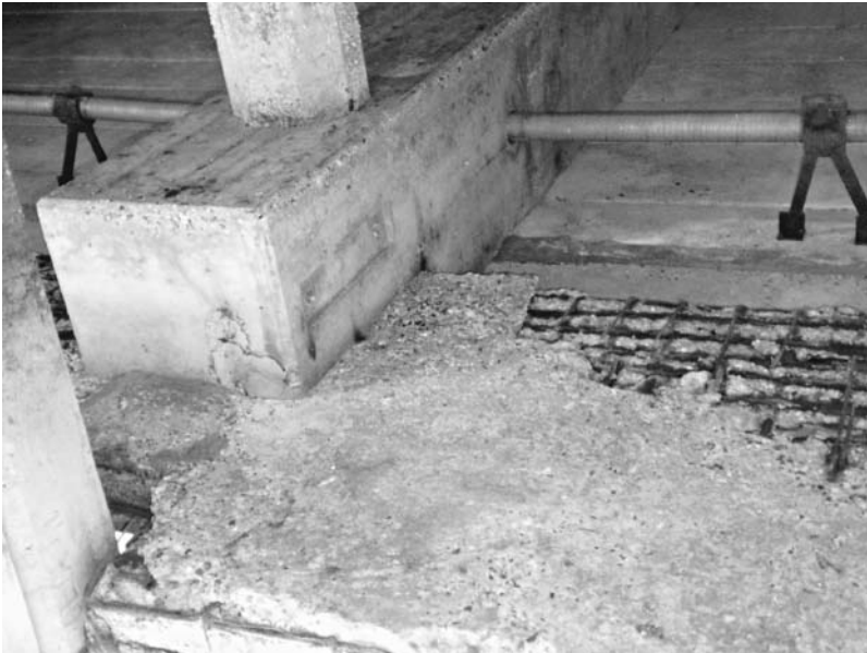
FIGURE 4.12 Example of corroded reinforcing steel in concrete quay, Kuwait.
