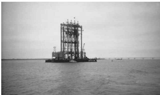
FIGURE 9.59 Mytilus densifying sands by intensive vibration.
