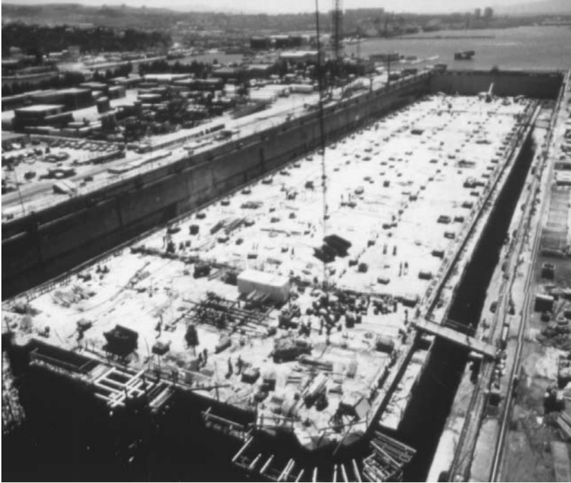
FIGURE 13.10 Completing construction of N'Kossa barge. (Courtesy of Buoygues Offshore.)
