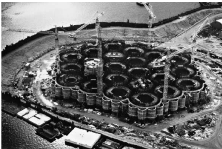
FIGURE 12.9 Base raft under construction.
