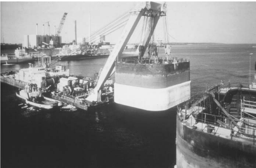
FIGURE 9.22 Concrete caisson for Great Belt Eastern Bridge, Denmark. Note attached cofferdam. (Courtesy of Great Belt Link Ltd.)
