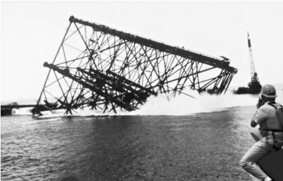
FIGURE 11.40 Launching of mid section of Cognac. (Courtesy of Shell Exploration and Production.)
