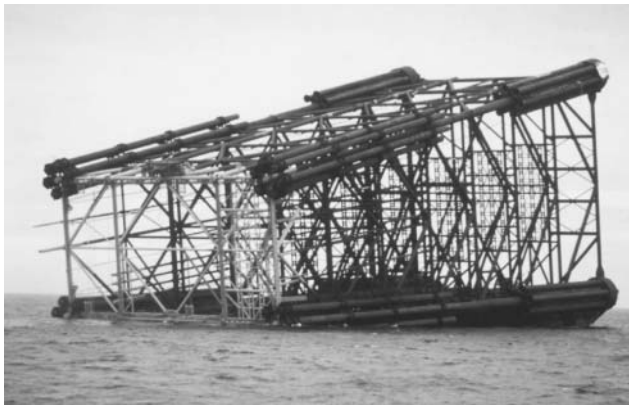
FIGURE 11.10 Commencing launch of platform Heather. (Courtesy of J. Ray McDermott, S.A.)
