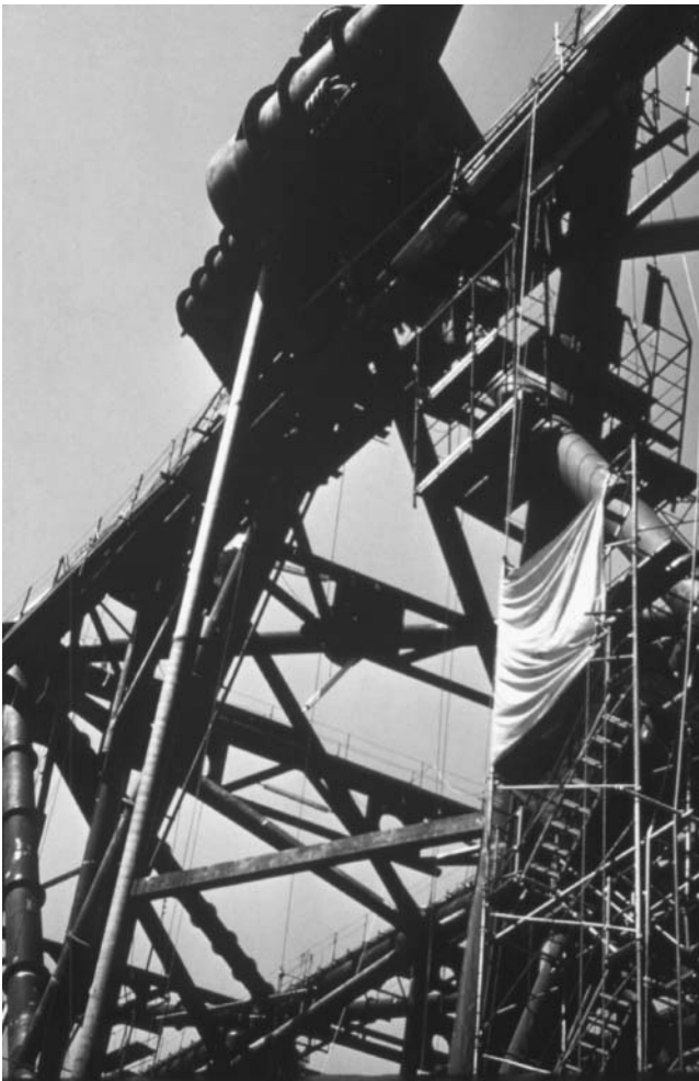
FIGURE 11.29 Male mating cone for Hondo jacket.
