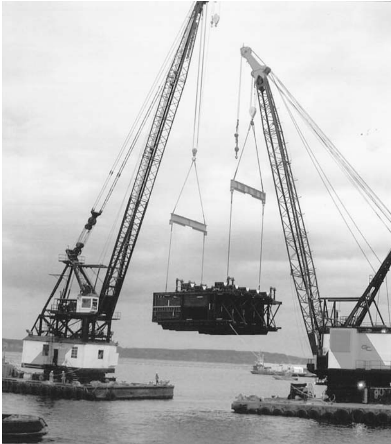
FIGURE 6.25 Setting Mooring Camel, Naval Base Bangor, Washington. (Courtesy of General Construction.)
