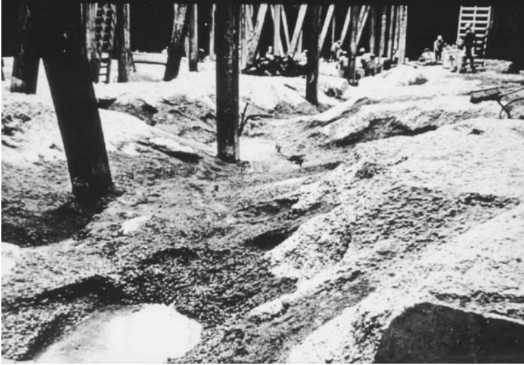
FIGURE 6.40 Failure of tremie concrete placement due to improper mix and placement.
