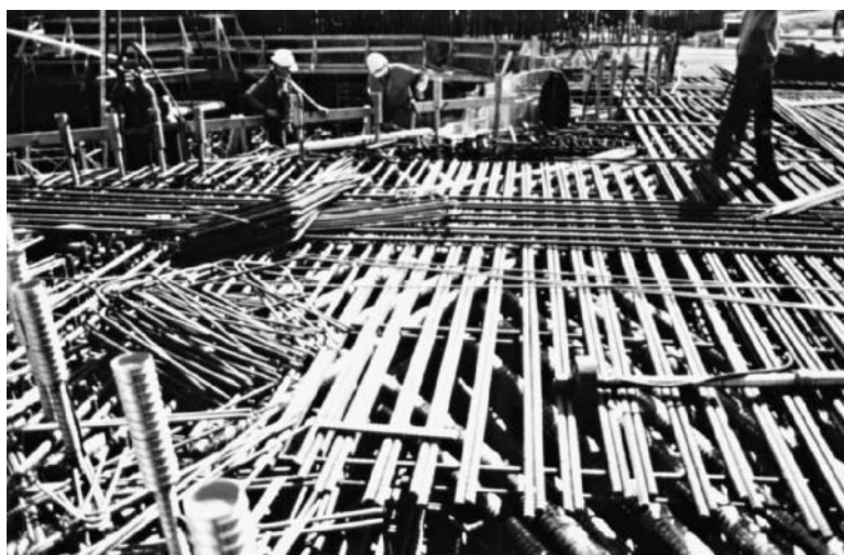
FIGURE 12.10 Ducts for post-tensioning tendons in base raft of Statfjord C.
