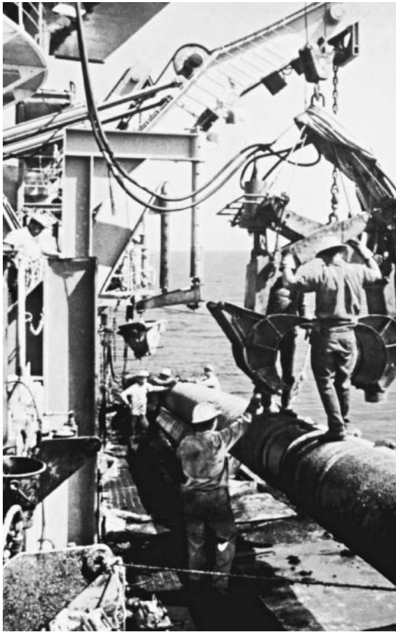
FIGURE 15.12 Coating the joint.
