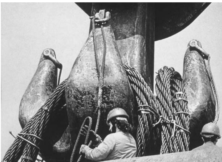
FIGURE 6.21 Hooking high capacity slings onto hook of heavy lift crane barge.
