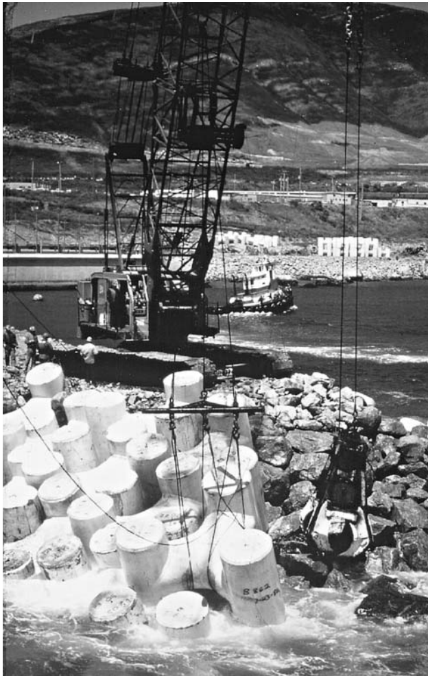
FIGURE 10.11 Precast armor units for breakwater.
