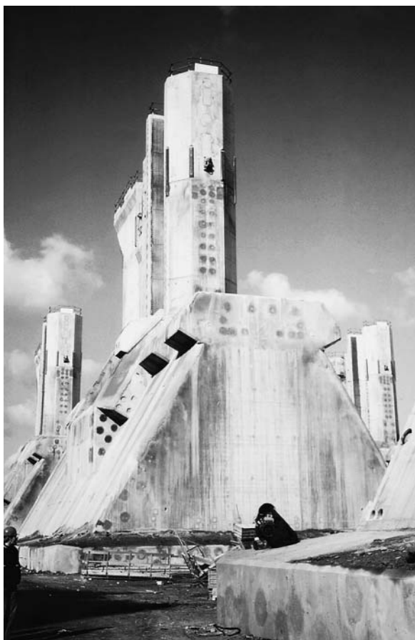
FIGURE 9.65 Prefabricated gate pier for Oosterschelde storm surge barrier.
