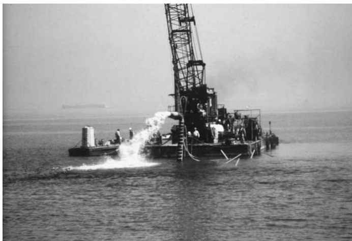
FIGURE 7.7 Large airlift pump excavating at a depth of 23 m.
