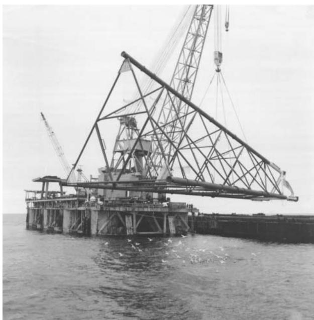
FIGURE 11.9 Lifting jacket with slings pre-attached. (Courtesy of Santa Fe International.)
