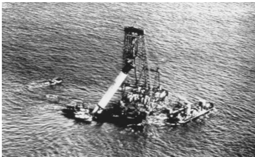
FIGURE 9.42 Upending concrete tubular pile for Oosterschelde Bridge.
