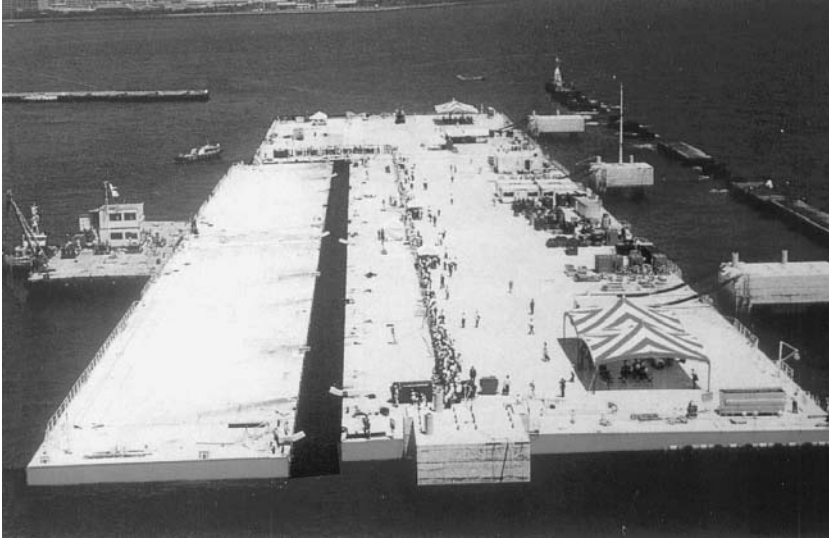
FIGURE 13.2 Mating of steel hulls for floating offshore base. Test of prototype.
