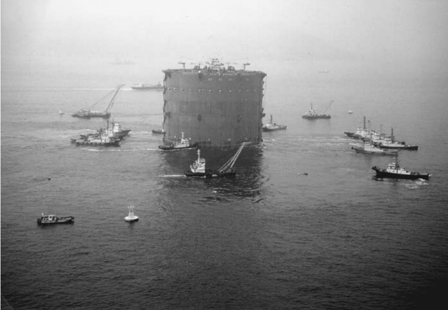
FIGURE 9.21 Steel caisson for main pier of Akashi Strait Bridge, Japan. (Courtesy of Kajima Engineering and Construction Co.)
