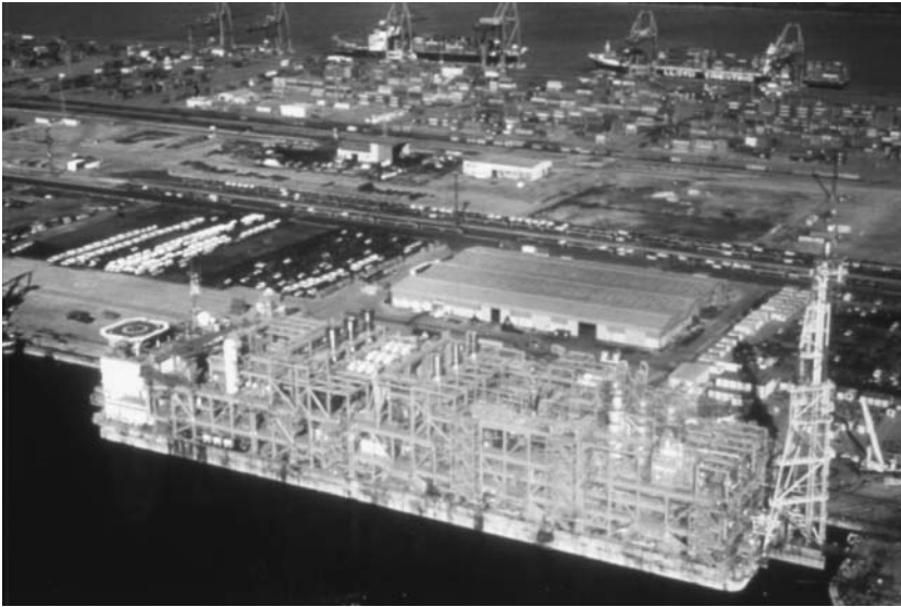
FIGURE 13.12 Installing superstructure and outfitting of N'Kossa barge. (Courtesy of Buoygues Offshore.)
