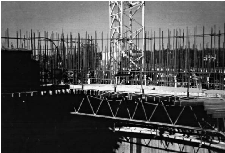
FIGURE 12.17 Slip-form construction of cell walls.
