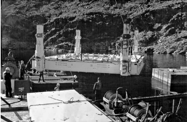
FIGURE 10.7 Frame for drilling template in deep water. (Courtesy of Southern Nevada Water District.)
