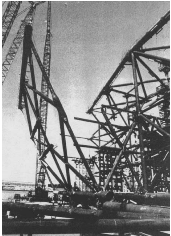
FIGURE 4.6 Roll-up of jacket framing. (Courtesy of Shell Exploration and Production.)
