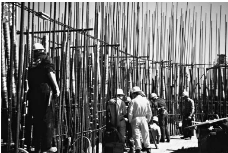
FIGURE 12.18 Extending reinforcing steel during slip forming.
