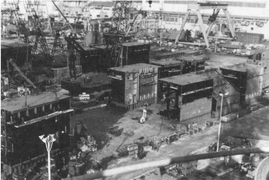
FIGURE 21.9 Japanese shipyard constructing steel base for Arctic offshore platform. Modular segments were shop-fabricated and joined in graving dock.
