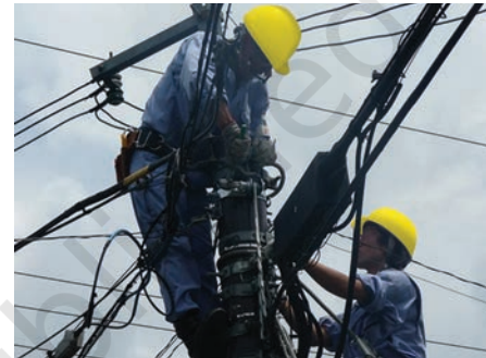
Fig. 4.53 Inspection of Power Distribution Lines
