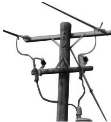
Fig. 4.15 Double-channel Cross-arms
