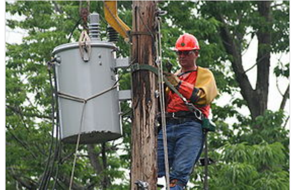
A lineman wearing equipment for hot glove work
