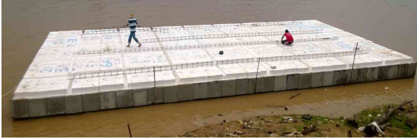
Fig. 8. Pontoon Modular EPS Source: B-Foam, 2017
