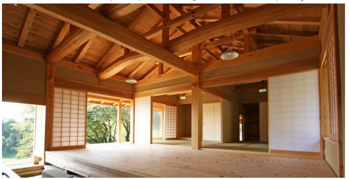
Wooden buildings are common for detached houses in Japan. They use a **post-and-beam system** for flexibility during earthquakes. Wood's **natural elasticity** helps absorb and dissipate seismic energy effectively.
