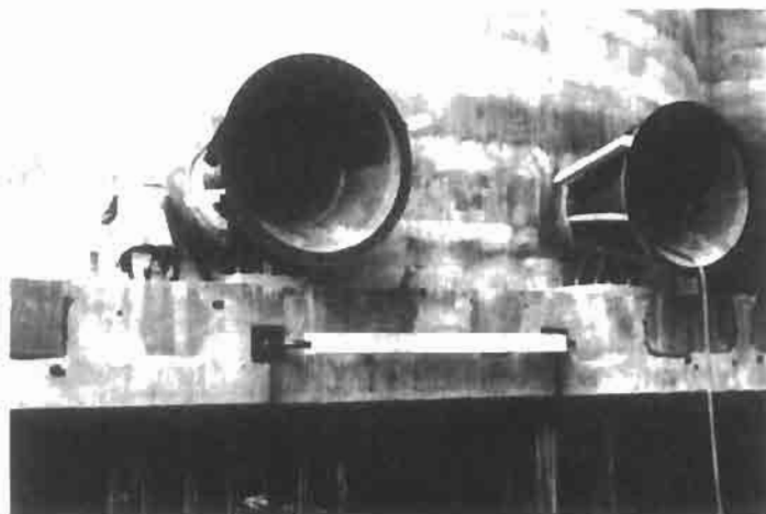
Fig. 16-6 Galvanic anodes on concrete structures.
