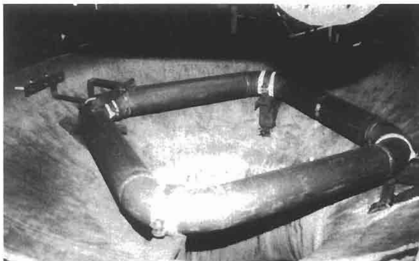
Fig. 21-12 Steel ring-shaped cathode in the heating chamber of a caustic evaporator.
