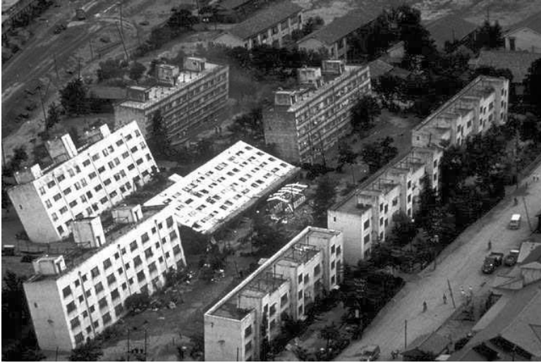
FIGURE 18.4 Liquefaction caused building failure in Niigata, Japan. (Photo by Joseph Penzien; photo courtesy of Steinbrugge Collection, Earthquake Engineering Research Center, University of California, Berkeley.)
