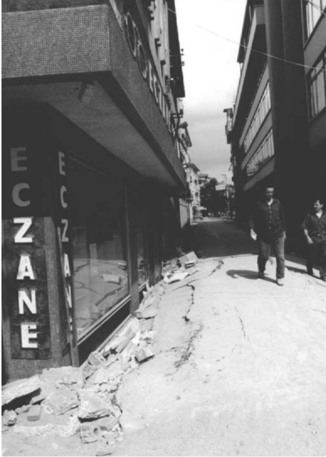
FIGURE 18.6 Settlement of building due to loss of bearing during the 1999 Kocaeli Earthquake.
