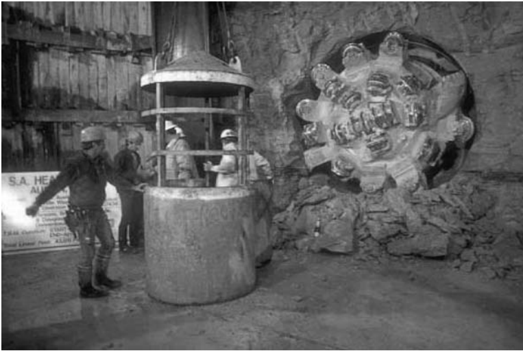
FIGURE 28.6 Rock TBM holing through (© David Sailors 1988, with permission).
