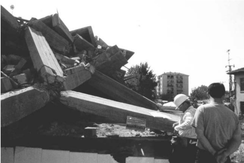
FIGURE 18.59 Collapsed reinforced concrete building during the 1999 Kocaeli Earthquake.
