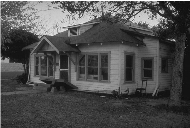
FIGURE 18.34 House that fell from its foundation during the 1971 San Fernando Earthquake. (Photograph courtesy of Steinbrugge Collection, Earthquake Engineering Research Center, University of California, Berkeley.)
