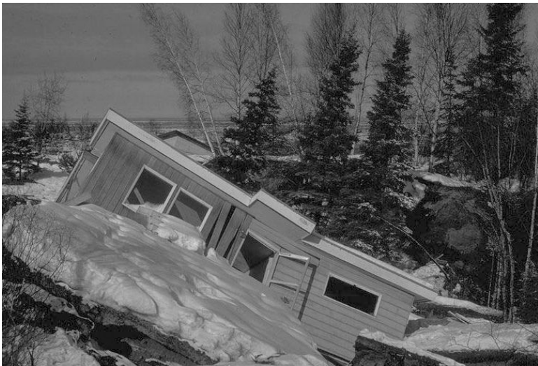
FIGURE 18.18 About 75 homes were damaged as a result of the Turnagain Heights Slide. (Photograph courtesy of Steinbrugge Collection, Earthquake Engineering Research Center, University of California, Berkeley.)
