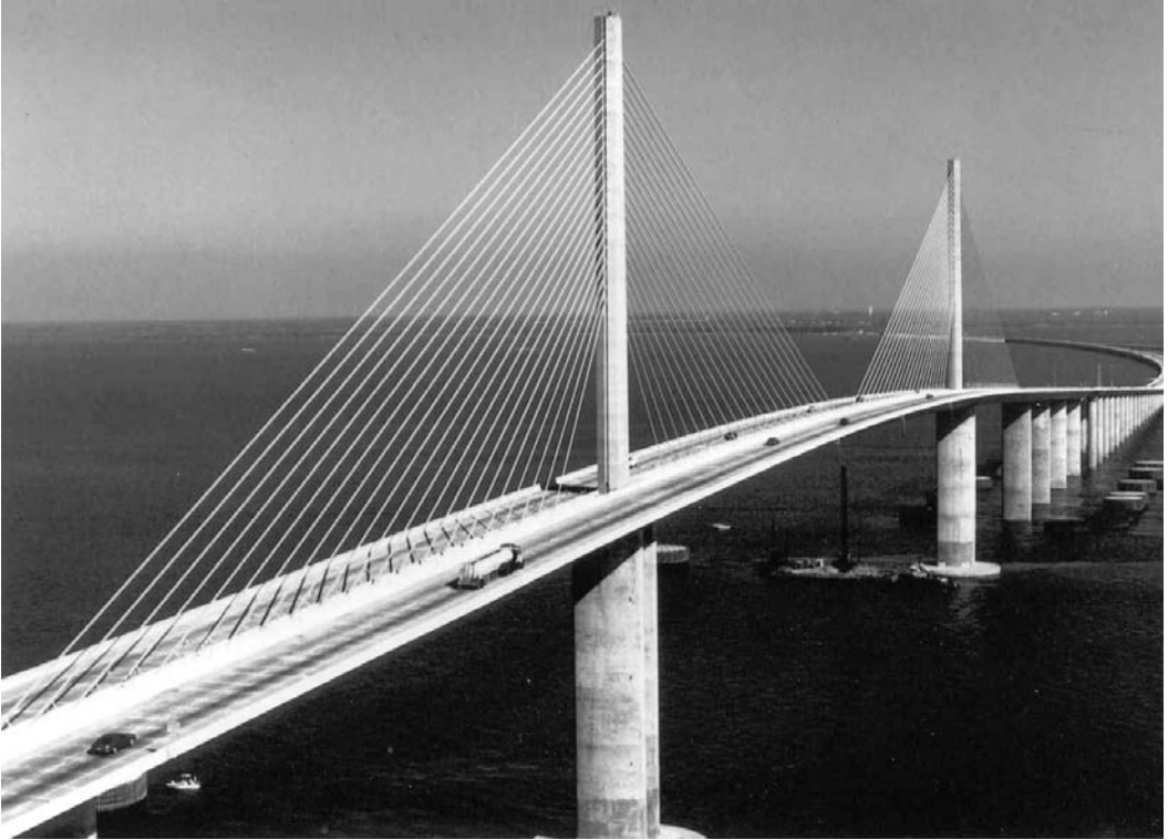
PHOTO 8.7 Sunshine Skyway Bridge, Tampa, Florida. Designed by Figg and Muller Engineers, Inc. The bridge has a 1200 ft cable-stayed main span with a single pylon, 175 ft vertical clearance, a total length of 21,878 ft and twin 40-ft roadways (courtesy Portland Cement Association).
