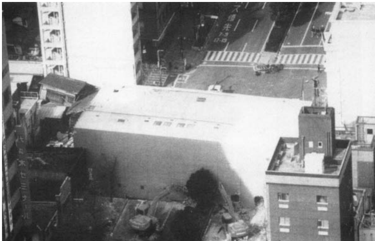
FIGURE 18.42 Eventual collapse of nine-story SRC building after the Kobe Earthquake. (Photo courtesy of NIST; NIST, The January 17, 1995 Hyogoken-Nanbu (Kobe) Earthquake, U.S. NIST, Gaithersburg, MD, 1996.)
