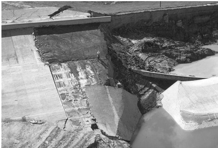
FIGURE 18.22 Closer view of damage to the Lower San Fernando Dam. (Photograph courtesy of Steinbrugge Collection, Earthquake Engineering Research Center, University of California, Berkeley.)
