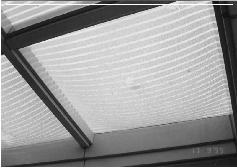
FIGURE 29.9 Laminated glass when it is broken.
