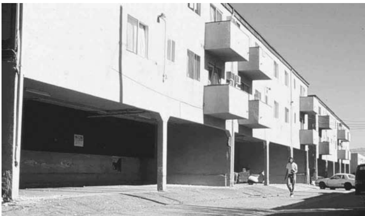
FIGURE 10.7 Typical soft story “tuck-under” parking, with apartments above (courtesy of EQE International).
