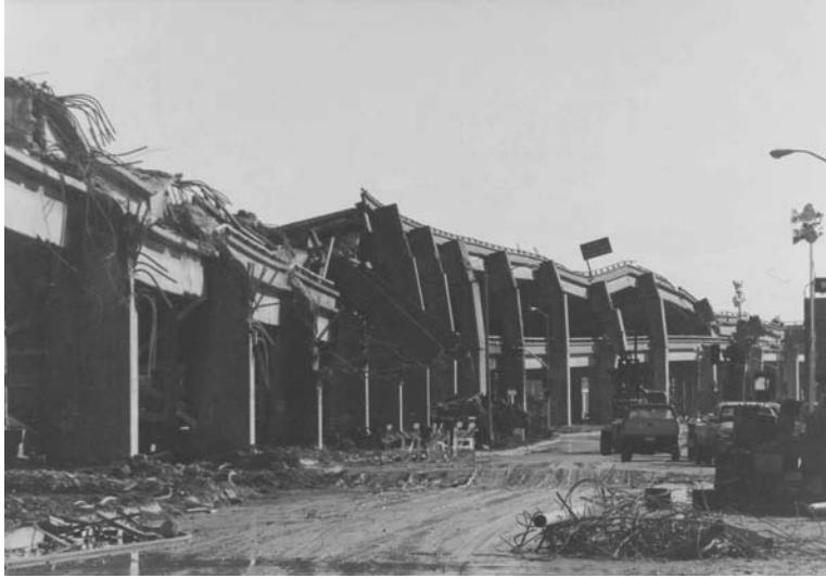
FIGURE 20.4 Collapse of Cypress Viaduct, California, in the 1989 Loma Prieta Earthquake.
