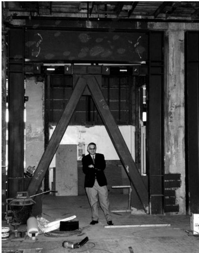
FIGURE 18.83 The steel frames included fluid viscous dampers to reduce the story drift. (Photo courtesy of Marr-Shaffer & Miyamoto, Structural Engineers.)
