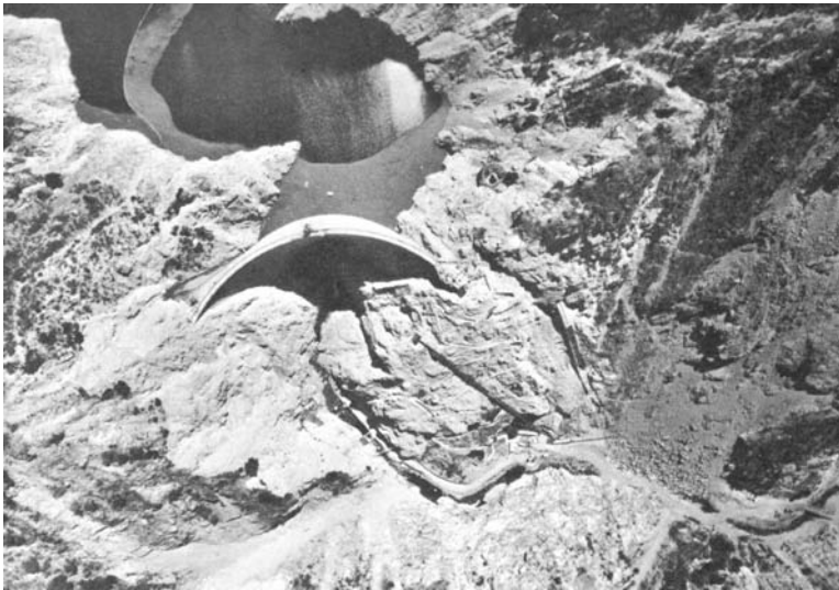
FIGURE 18.20 Landslides at Pacoima Dam following the 1971 San Fernando Earthquake. (Photograph courtesy of Steinbrugge Collection, Earthquake Engineering Research Center, University of California, Berkeley.)
