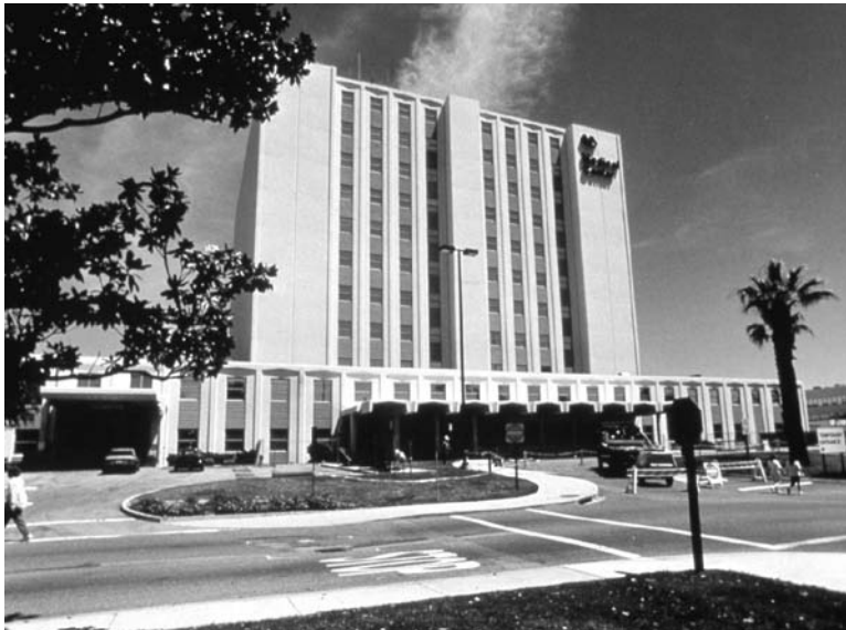
FIGURE 18.84 The existing Long Beach VA Hospital was seismically retrofit with lead-rubber bearings. (Photo courtesy of Dynamic Isolation Systems, Inc.)
