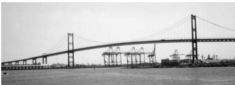
FIGURE 18.87 The Vincent Thomas Bridge is a three-span suspension structure built over the port of Los Angeles.
