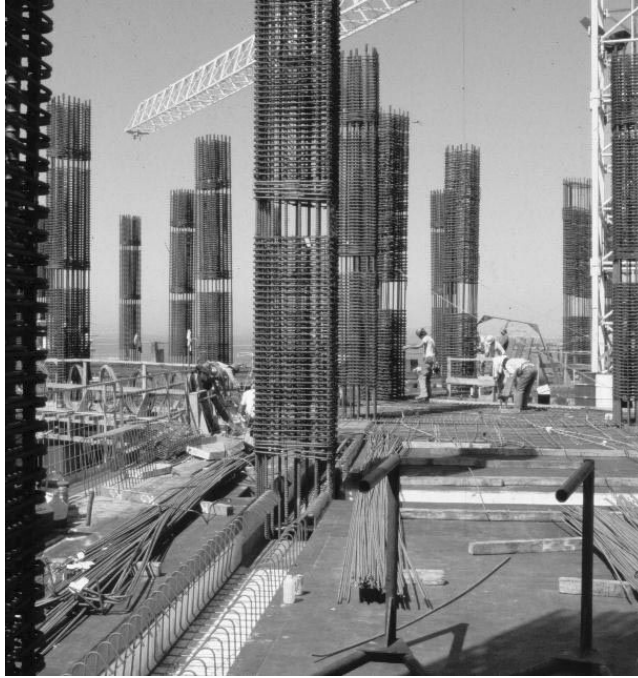
PHOTO 7.2 Installation of reinforcing bars in the Pacific Park Plaza building (courtesy of Mr. James Tai, T.Y. International, San Francisco).
