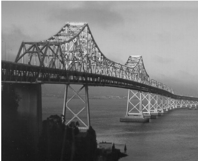
FIGURE 25.6 San Francisco-Oakland Bay Bridge — east span.
