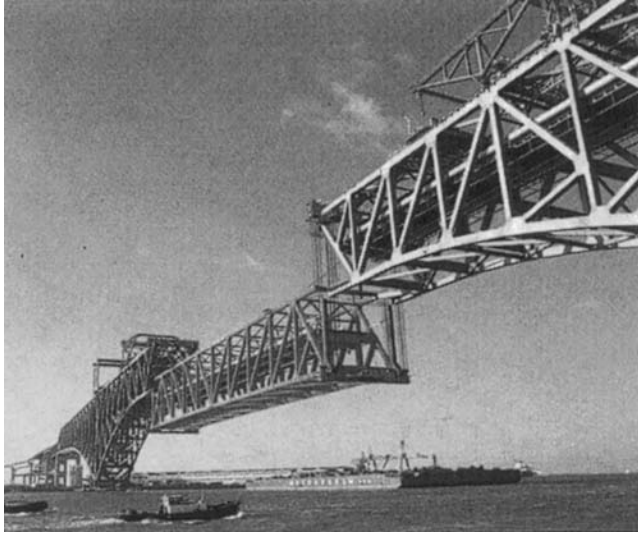
FIGURE 25.46 Lifting erection of Minato Oh-Hashi, Japan (Gerber bridge 1974) (HEPC 1994).
