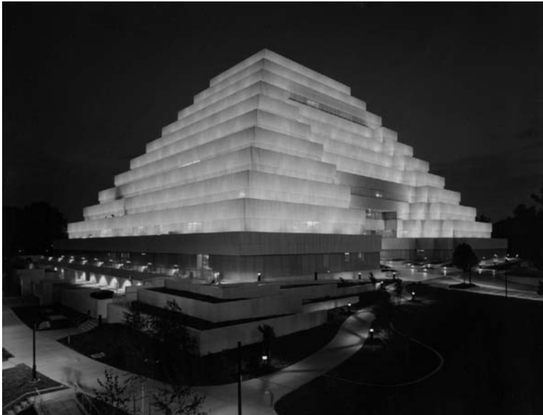
FIGURE 18.81 The uniquely shaped “Money Store” was designed with fluid viscous dampers to improve its seismic behavior. (Photo courtesy of Marr-Shaffer & Miyamoto, Structural Engineers.)
