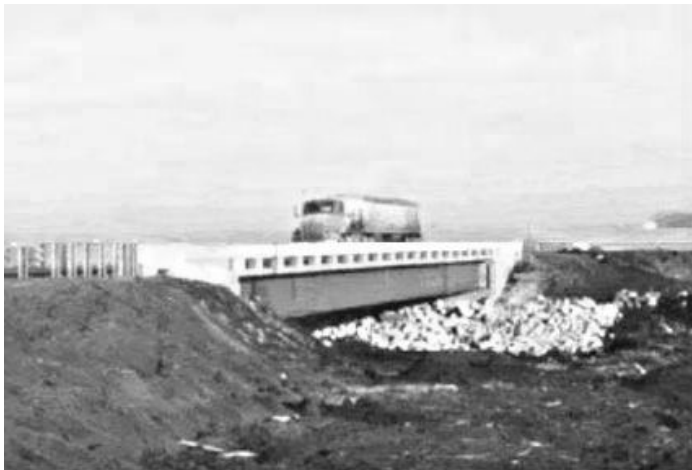
FIGURE 14.2 Snyder South Bridge (courtesy of Nebraska DOT and FHWA).
