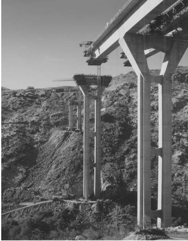
FIGURE 25.37 Pine Valley Bridge — construction stage, California.
