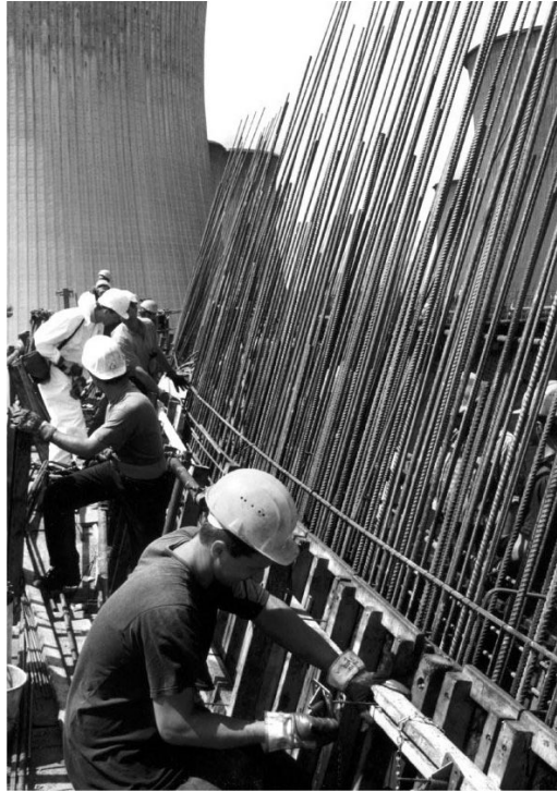
FIGURE 27.7 Formwork and steel reinforcement of shell wall.
