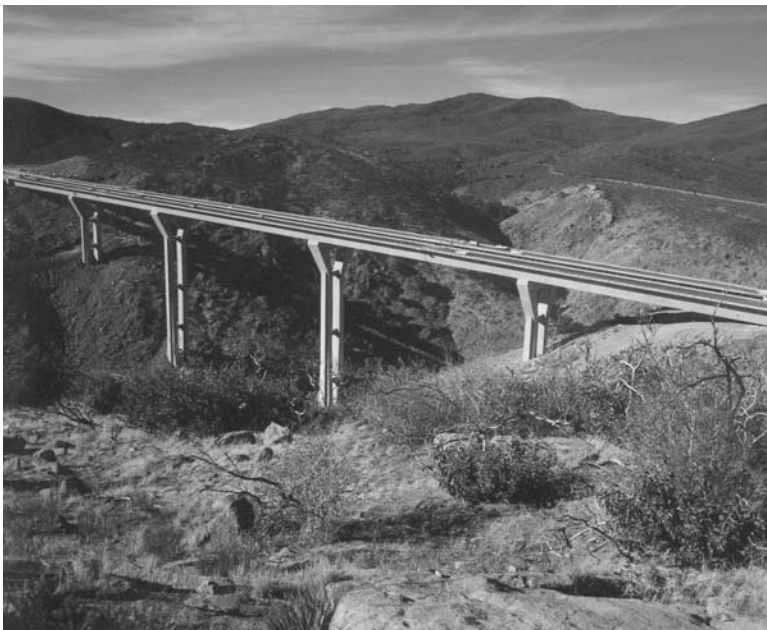
FIGURE 25.38 Pine Valley Bridge — construction completed, California.
