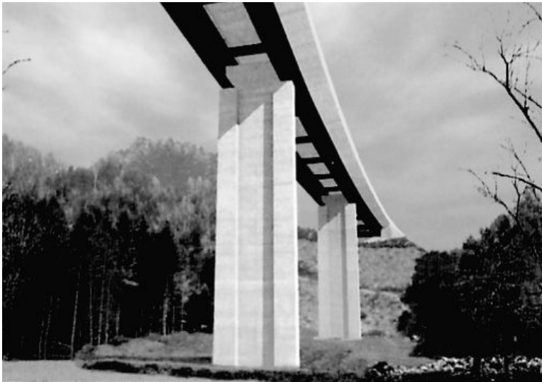
FIGURE 25.23 Widely spaced girder bridge (Chidorinosawagawa Bridge, Japan, from Kawasaki Heavy Ind., Ltd., with permission).
