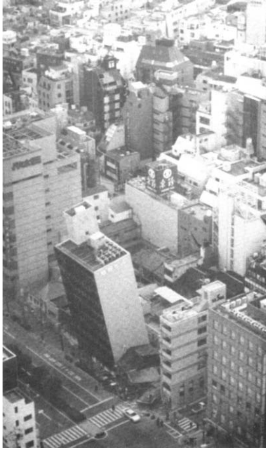
FIGURE 18.41 Nine-story SRC building immediately after the 1995 Kobe Earthquake. (Photo courtesy of NIST; NIST, The January 17, 1995 Hyogoken-Nanbu (Kobe) Earthquake, U.S. NIST, Gaithersburg, MD, 1996.)
