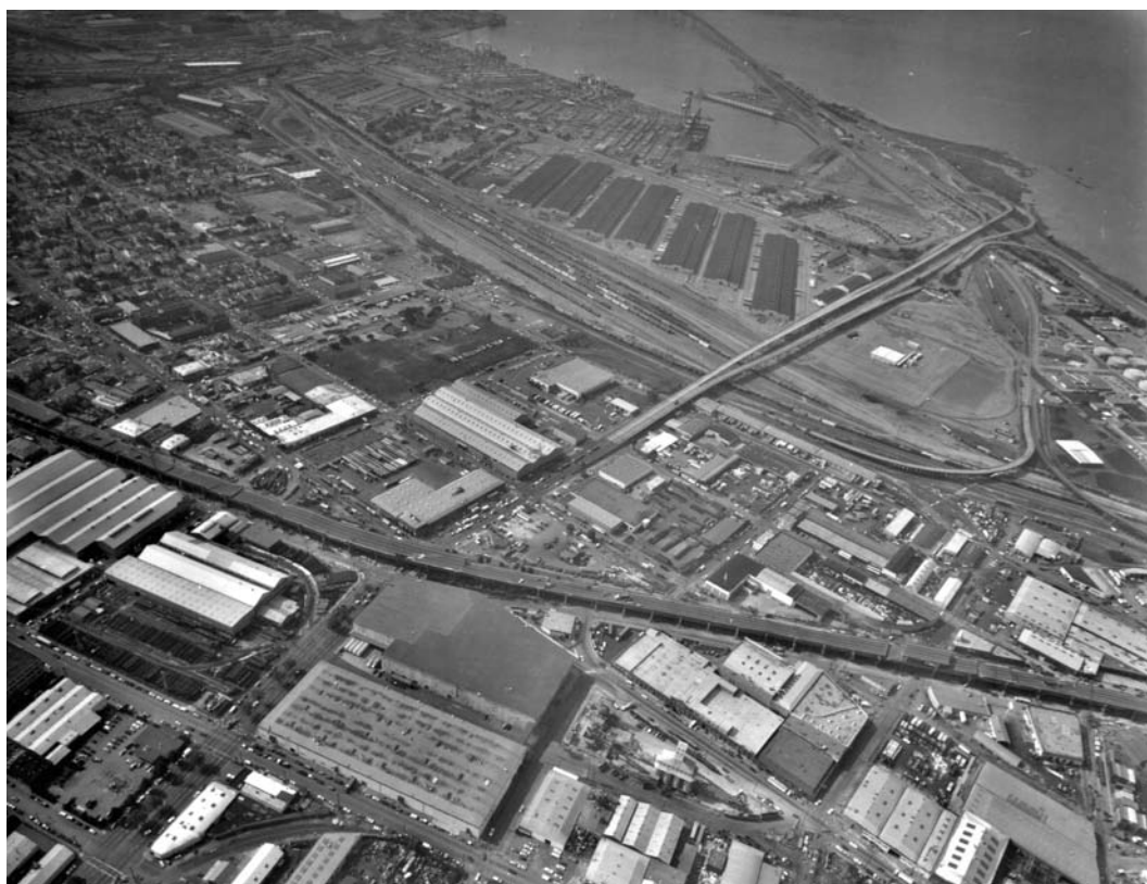
FIGURE 18.29 Aerial view of Cypress Viaduct showing collapse where the structure crossed over Bay mud.
