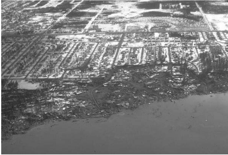
FIGURE 18.17 Aerial view of Turnagain Slide. (Photograph courtesy of Steinbrugge Collection, Earthquake Engineering Research Center, University of California, Berkeley.)
