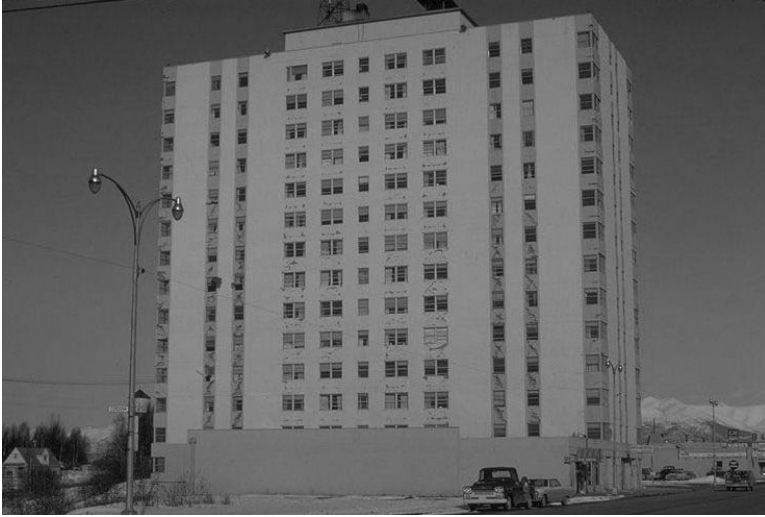
FIGURE 18.48 West elevation of the Mt. McKinley Apartment building after the 1964 Great Alaska Earthquake. (Photograph by Karl Steinbrugge, Earthquake Engineering Research Center, University of California, Berkeley.)
