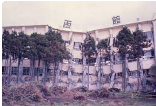
Damage from the 1968 Tokachi Earthquake: Collapsed Building in Japan
