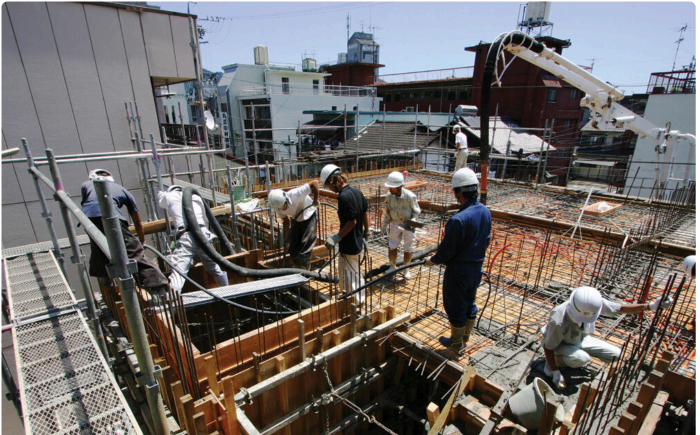
Construction site of a Reinforced Concrete (RC) Building in Japan
