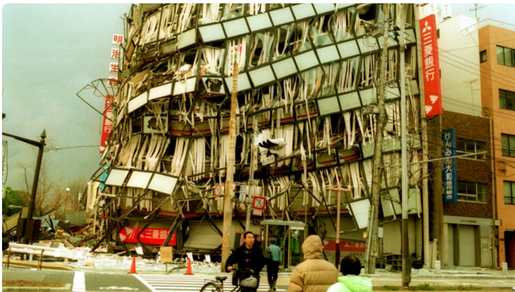
Collapsed Mitsubishi Bank Hyogo Branch Building following the Great Hanshin-Awaji Earthquake in 1995
