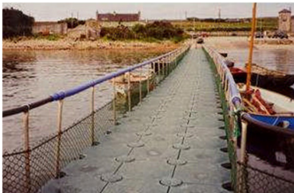
Figure 2. Commercial floating pontoon.
