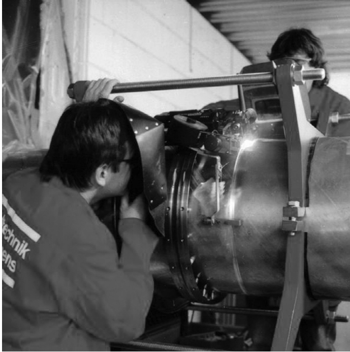
FIGURE 18.17 Computer-controlled orbital welding on site. (Courtesy of Siemens.)
