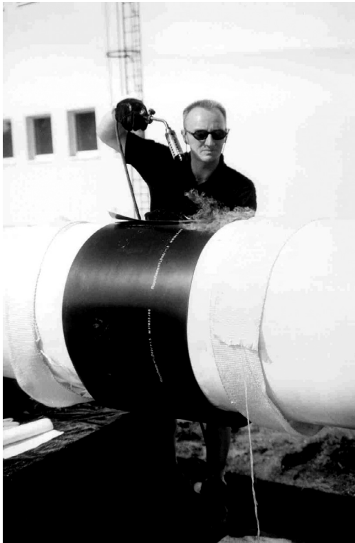
FIGURE 18.29 On-site corrosion protection of the welding area—shrinking method. (Courtesy of Siemens.)
