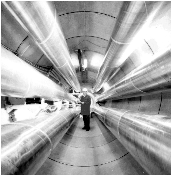
FIGURE 18.7 View into the tunnel. (Courtesy of Siemens.)
