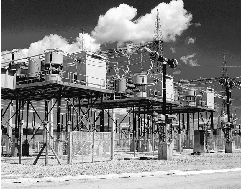
FIGURE 5.15 TCSC Serra da Mesa, FURNAS, Brazil, 500 kV, 107 MVar, (1 \dots 3) \times 13.17 W. (Photo courtesy of Siemens.)
