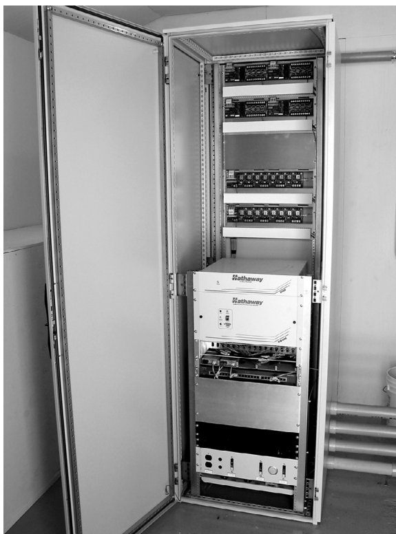
FIGURE 7.6 Secondary substation integration and automation system.
