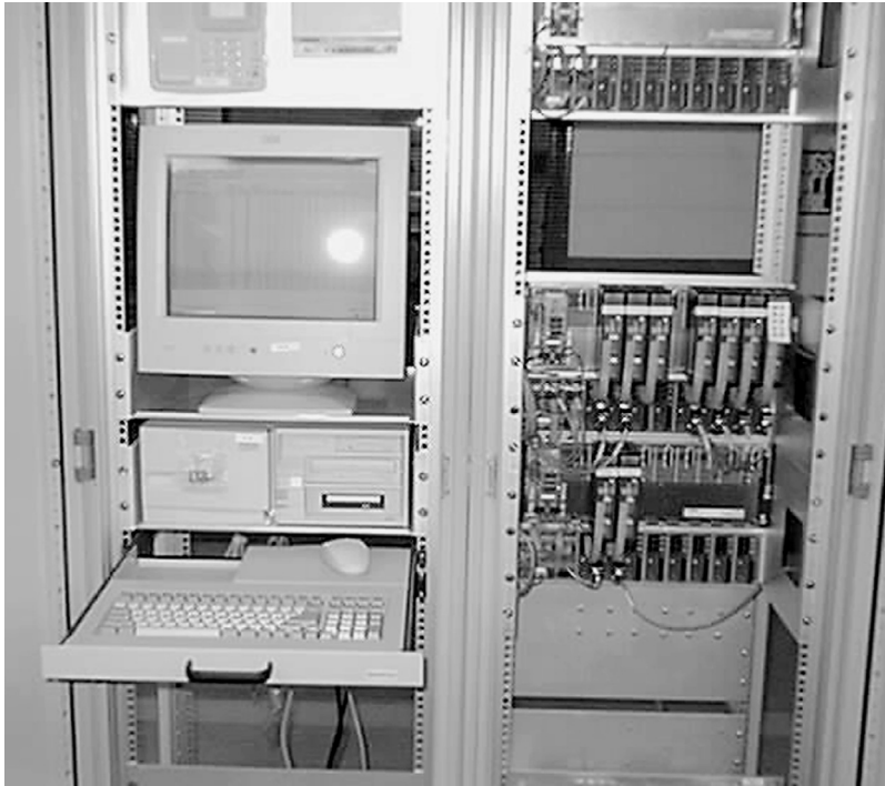
FIGURE 7.2 Substation automation system.
