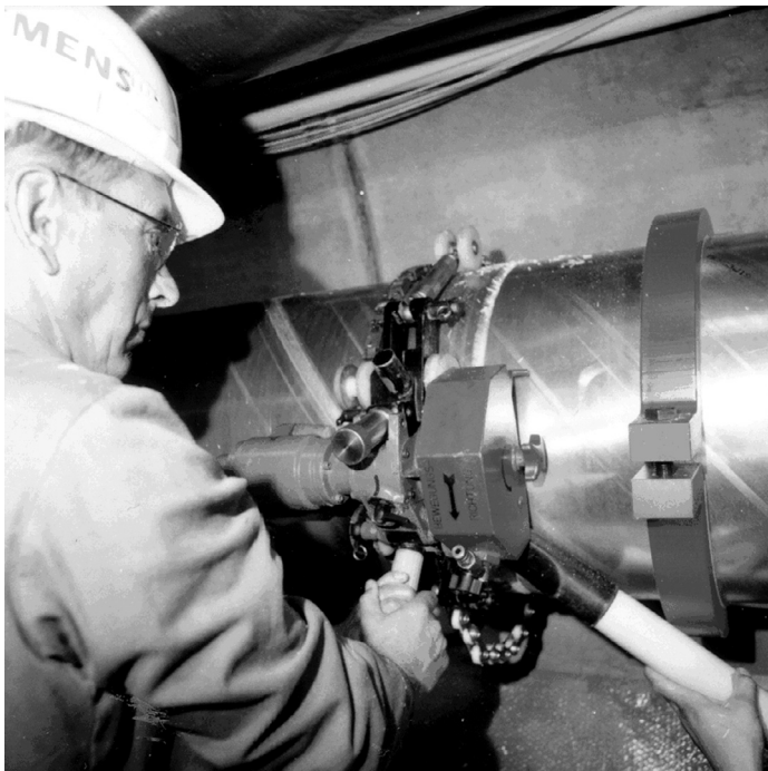
FIGURE 18.18 Cutting the enclosure pipe with a saw. (Courtesy of Siemens.)
