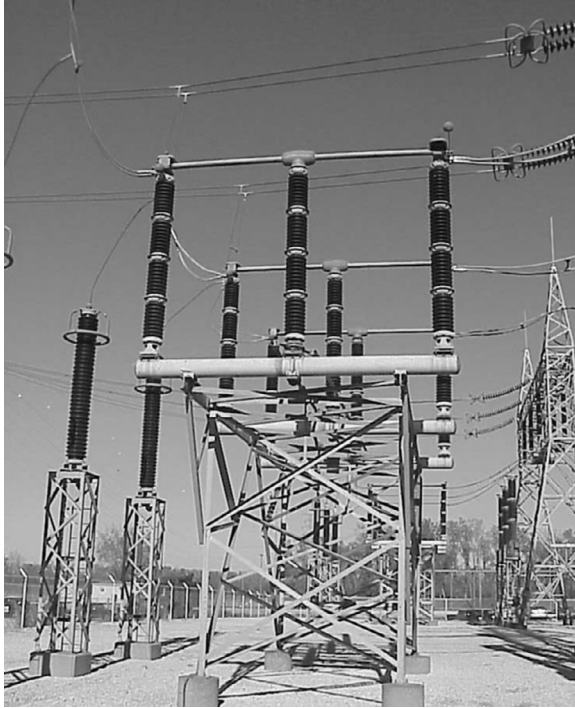
FIGURE 4.12 Double end break (double side break) disconnect switch.
