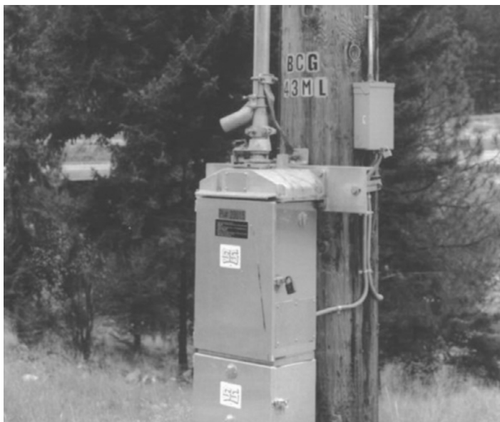
FIGURE 4.7 Stored energy motor operator for disconnect switch.
