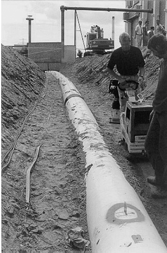
FIGURE 18.6 Banded tube and backfilling. (Courtesy of Siemens.)
