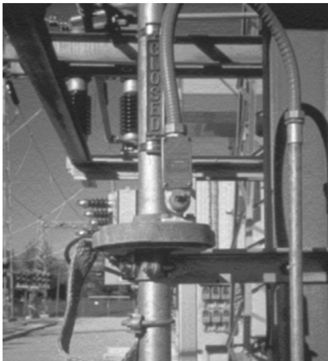
FIGURE 4.2 Key type interlock.
