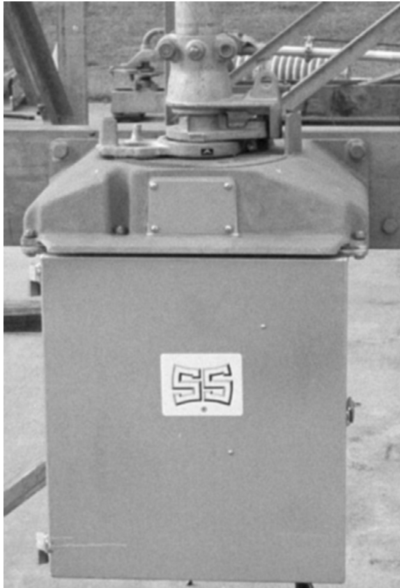
FIGURE 4.6 Motor operator for disconnect switch.
