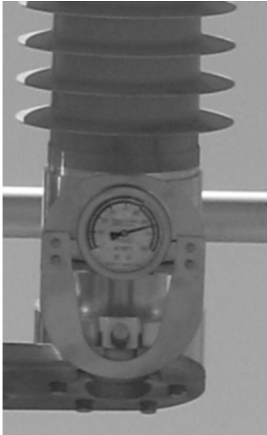
FIGURE 4.29 SF 6 interrupter's pressure indicator.
