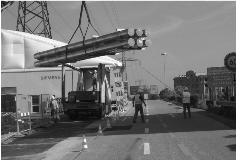
FIGURE 18.26 Delivery of transport unit to the preassembly area. (Courtesy of Siemens.)
