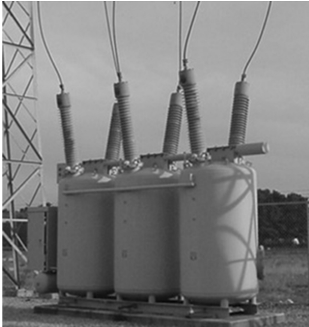
FIGURE 4.39 Three tank bulk oil circuit breaker.
