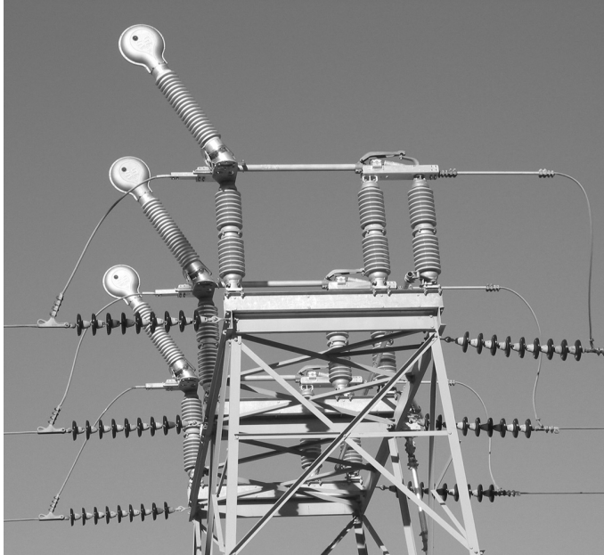
FIGURE 4.27 Load break switch with SF 6 interrupters.
