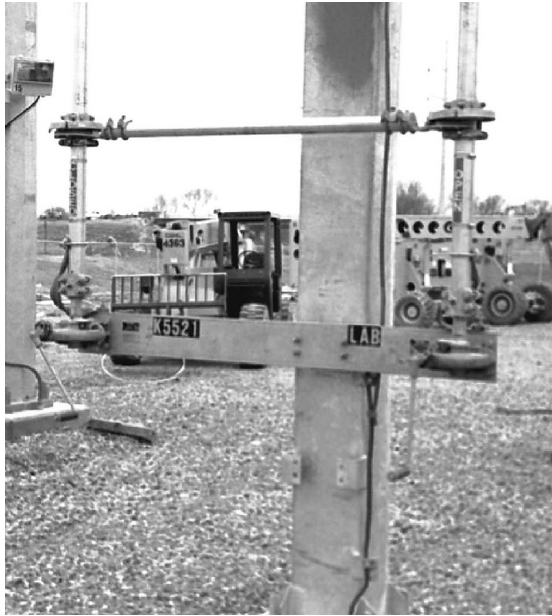
FIGURE 4.1 Mechanical cam-action type interlock.
