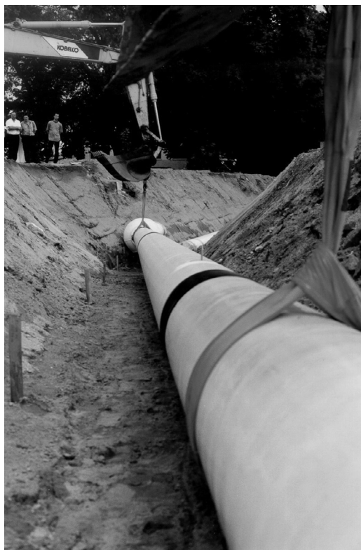
FIGURE 18.5 Laying the GIL into the soil. (Courtesy of Siemens.)
