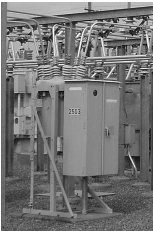
FIGURE 4.38 Single tank bulk oil circuit breaker.
