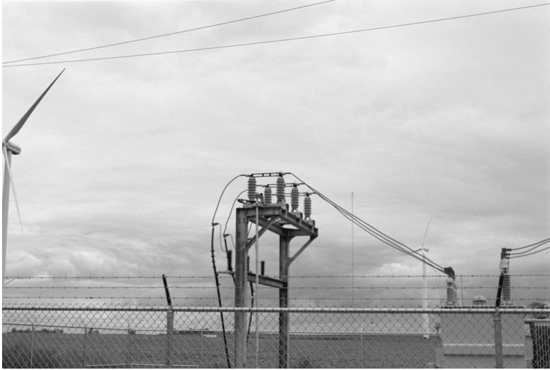
FIGURE 4.16 Single side break disconnect switch.
