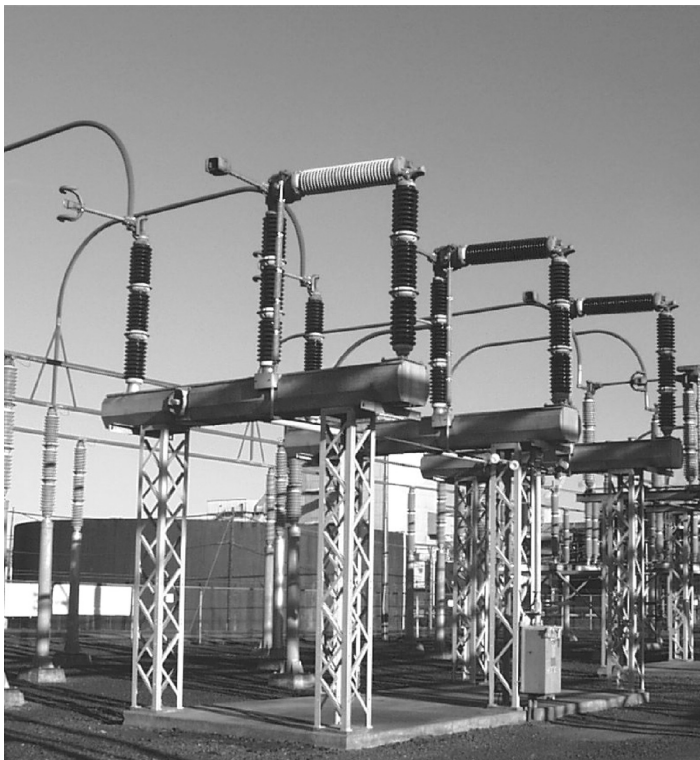
FIGURE 4.33 Multiple interrupter gap per phase circuit switcher.
