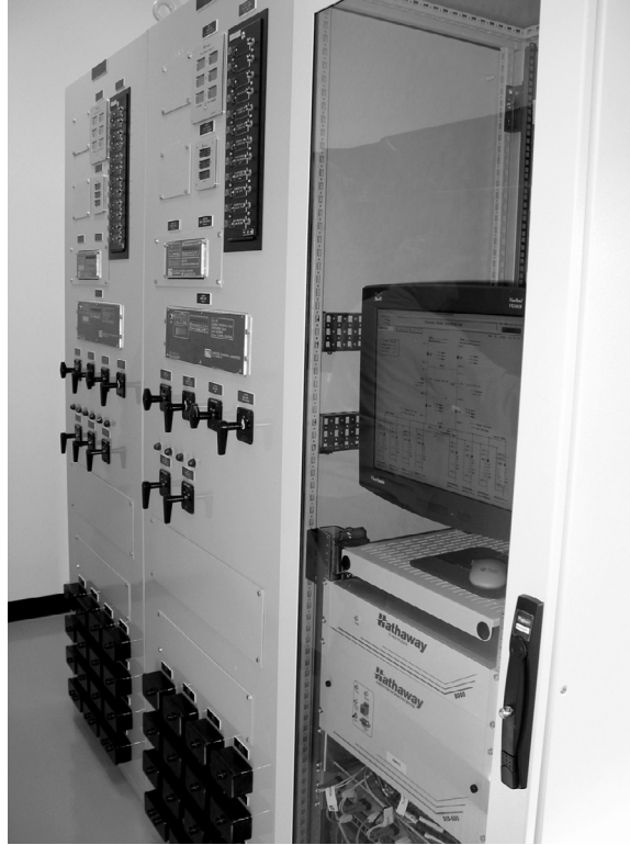
FIGURE 7.5 Primary substation integration and automation system.
