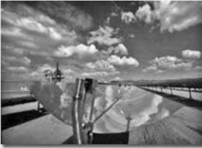
Figure 5.3 The Concentrated Parabolic Trough Solar Power System. 6 (Photo courtesy of the California Energy Commission)
