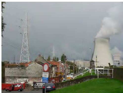
Figure 32.24 The people living near this nuclear power plant have no measurable exposure to radiation that is traceable to the plant. About 16% of the world's electrical power is generated by controlled nuclear fission in such plants. The cooling towers are the most prominent features but are not unique to nuclear power. The reactor is in the small domed building to the left of the towers. (credit: Kalmthouts)
