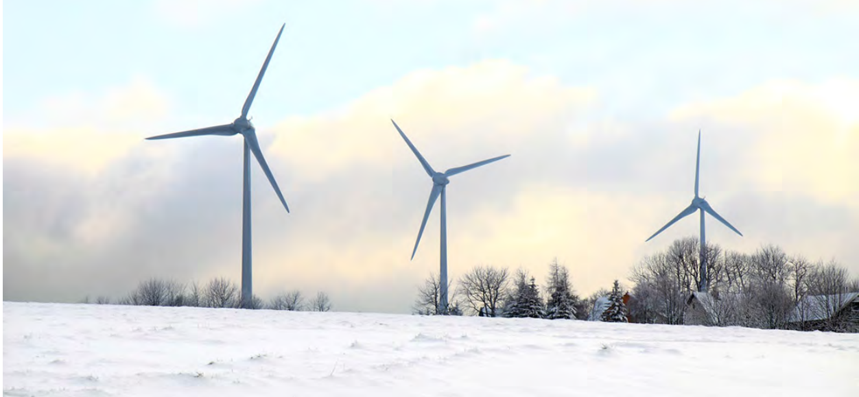
Figure 23.1 These wind turbines in the Thames Estuary in the UK are an example of induction at work. Wind pushes the blades of the turbine, spinning a shaft attached to magnets. The magnets spin around a conductive coil, inducing an electric current in the coil, and eventually feeding the electrical grid. (credit: modification of work by Petr Kratochvil)
