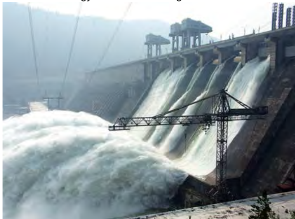
Figure 7.38 Hydroelectric facility (credit: Denis Belevich, Wikimedia Commons)
