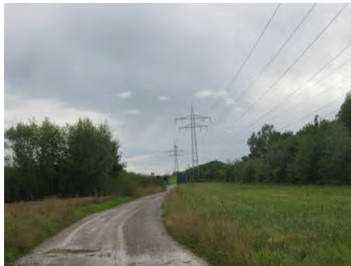
Figure 24.10 This high-voltage traction power line running to Eutingen Railway Substation in Germany radiates electromagnetic waves with very long wavelengths. (credit: Zonk43, Wikimedia Commons)
