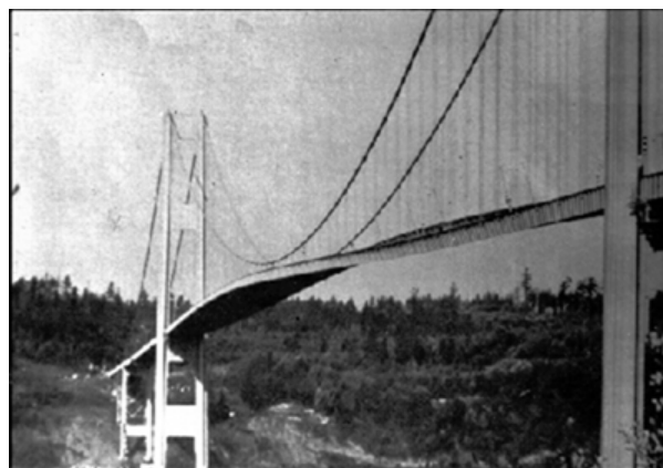
Figure 16.28 In 1940, the Tacoma Narrows Bridge in Washington state collapsed. Heavy cross winds drove the bridge into oscillations at its resonant frequency. Damping decreased when support cables broke loose and started to slip over the towers, allowing increasingly greater amplitudes until the structure failed (credit: PRI's Studio 360 , via Flickr)
