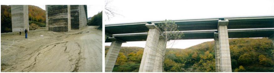
**Fig. 1.34** Fault trace running across the Bolu Viaduct piers (*left*) and the damage caused at the deck structure due to static differential movement of the piers along the ruptured fault
