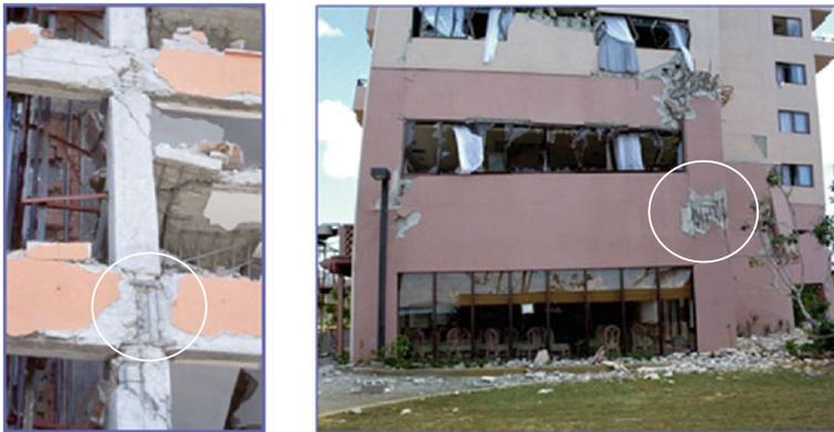
**Fig. 7.23** Joint failures observed in non-ductile reinforced concrete buildings due to strong ground shaking (from Moehle et al. 2004)
