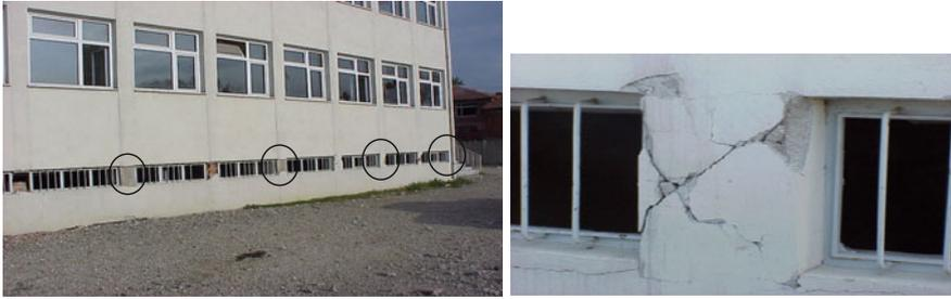
**Fig. 7.19** Short column failures in a school building after the 1999 Düzce earthquake. Picture on the right shows detailed shear damage from one of the short columns
