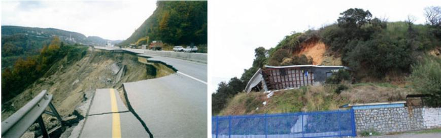
**Fig. 1.38** Landslide at a highway embankment during the 1999 Düzce earthquake (*left panel*) and landslide directly above structure during the 2010 Maule, Chile earthquake (*right panel*, EERI Earthquake Photo Gallery)
