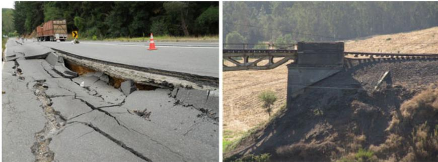
**Fig. 1.35** Ground failure in a highway (*left panel*) and extensive settlement in a railroad bridge abutment (*right panel*) during the 2010 Maule, Chile earthquake (EERI Earthquake Photo Gallery)
