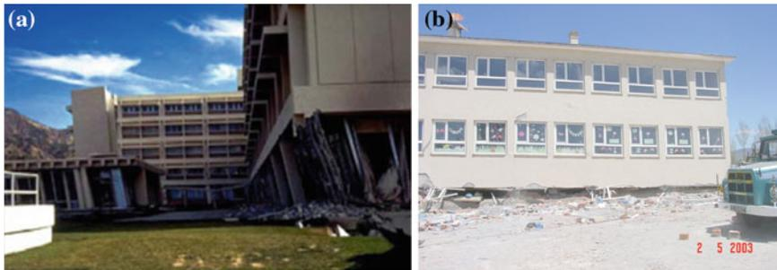
**Fig. 7.15** Soft story collapses from a 1971 San Fernando Earthquake, USA on the left, b 2003 Bingöl earthquake, Turkey on the right
