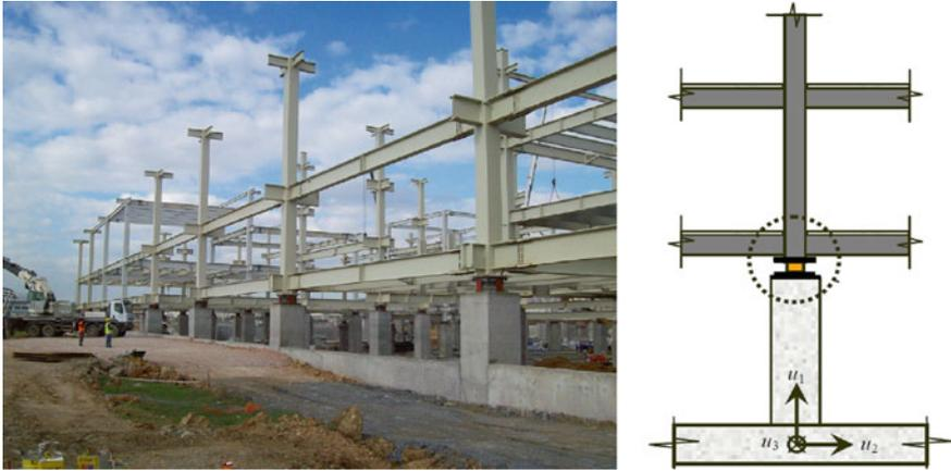
**Fig. 5.17** Base isolation interface between concrete basement and steel upper structure of a building
