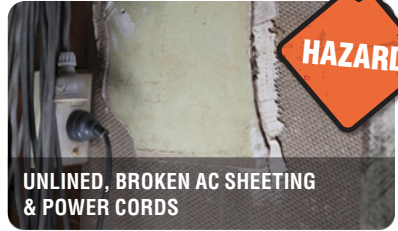
ASBESTOS WARNING ON POWER BOARD
