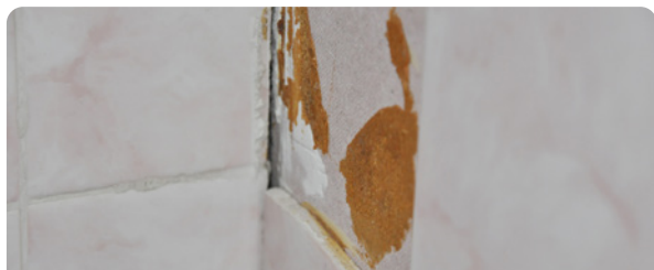
TILES & WALLS: GLUE AND BACKING BOARD
