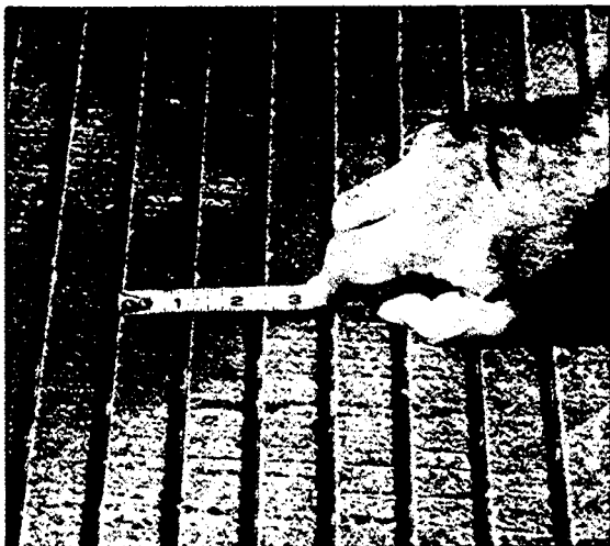
FIGURE 9-63. Cross cutting runways reduces danger of hydroplaning.
